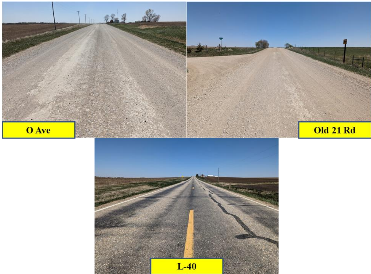
Figure B1. Otta seal site appearance in Cherokee County (photos taken on May 3, 2023)
