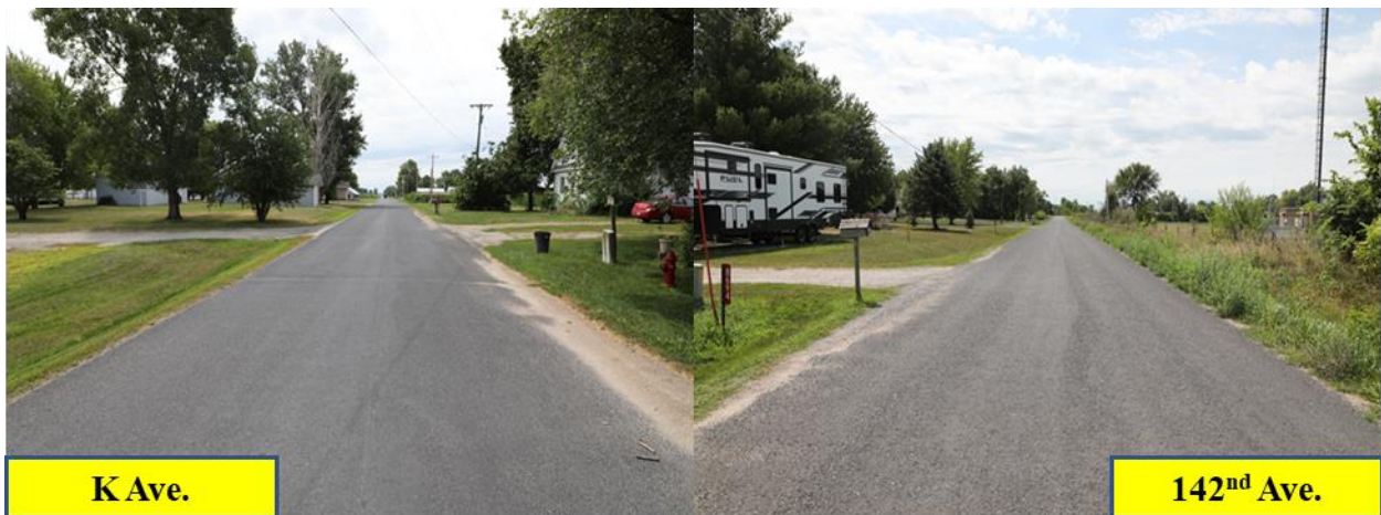
Figure B3. Otta seal site appearance in Louisa County (photos taken on July 31, 2023).
