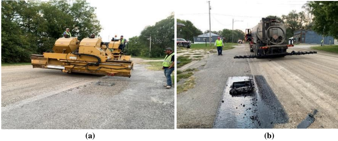
Figure 34. Calibration of equipment prior to Otta seal application: (a) adjusting aggregate application rate and (b) adjusting binder application rate
