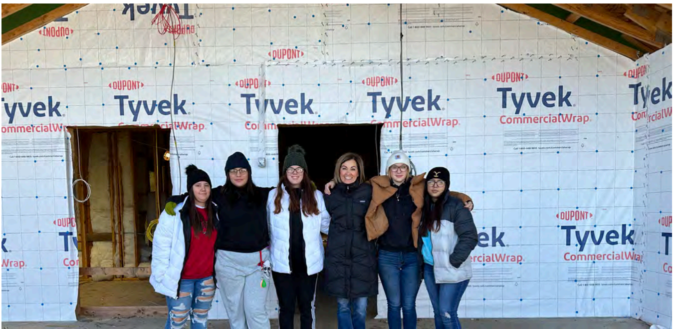
Gov. Reynolds tours the Ember Youth Recovery Campus construction site on Nov. 11, 2023.
