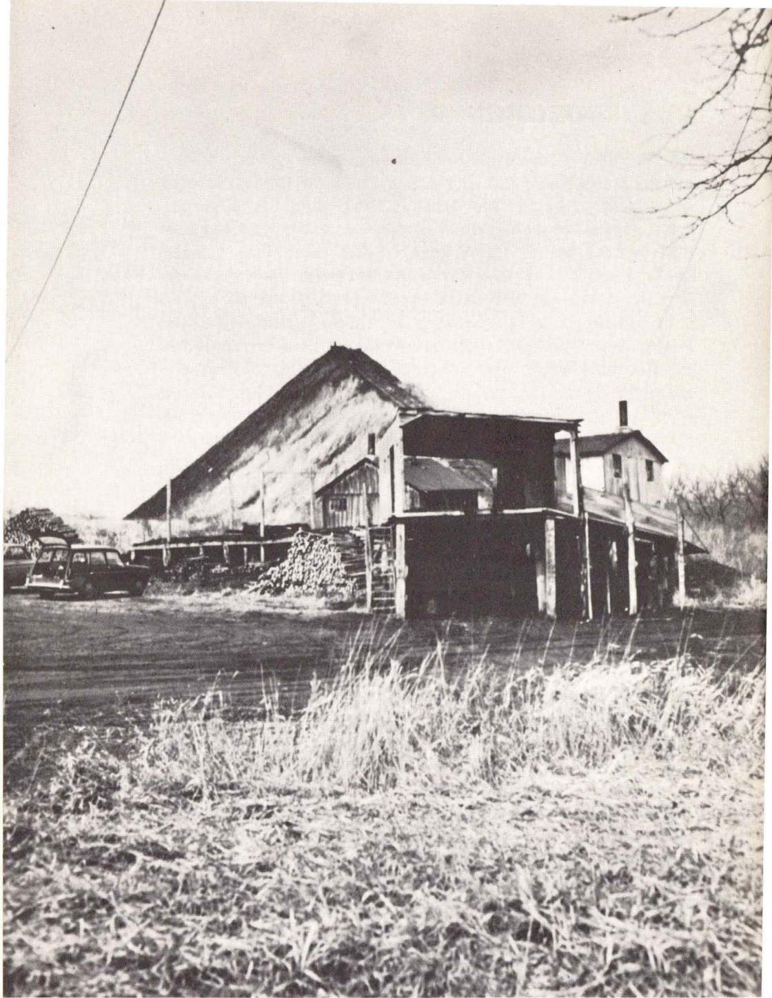
A topside view of the New Gladstone mine. The headhouse is at the right and the dumping platform is in the foreground. Dirt piles like the one in the background are reminders of the many coal mines that once operated in the area. (Photo courtesy Coal Mining and Processing .)
