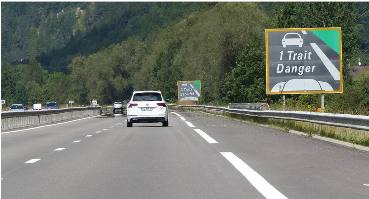
Figure 1. Anti-tailgating edge line markings and signage on Autoroute A40 in Magland, Haute-Savoie, France, 2017, with signs reading “1 Stripe Danger, 2 Stripes Safety”
