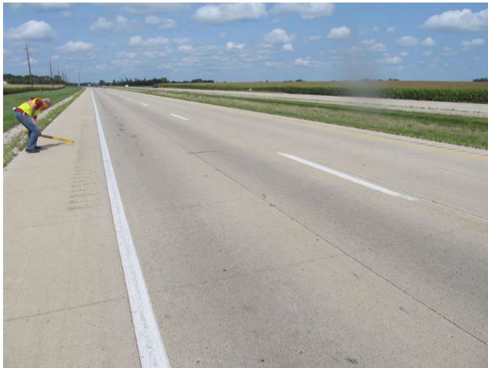
Shoulder cross slope 3.3%, Design 4%.
