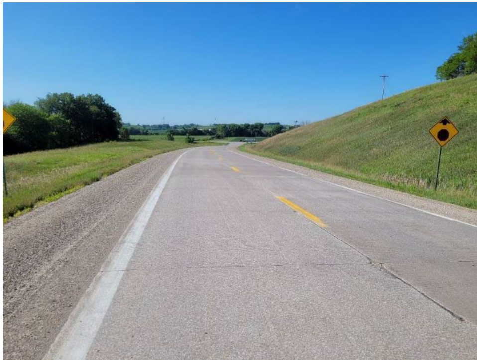
Figure 2 – 6-inch Overlay 12 x 12 ft. Joint Spacing
