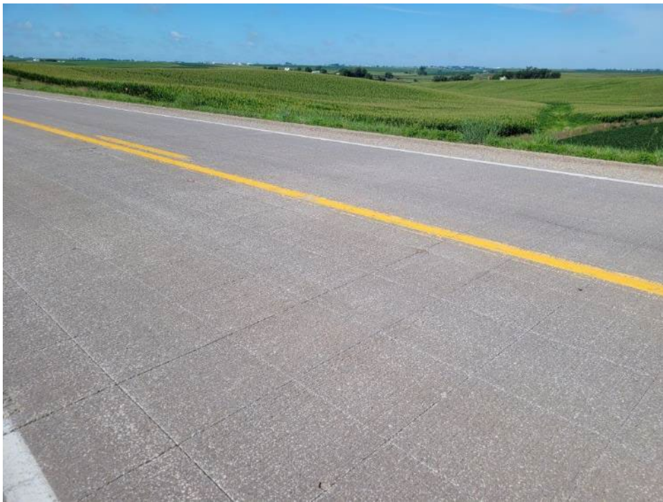
Figure 6 – 4-inch overlay 2 x 2 ft. Joint Spacing
