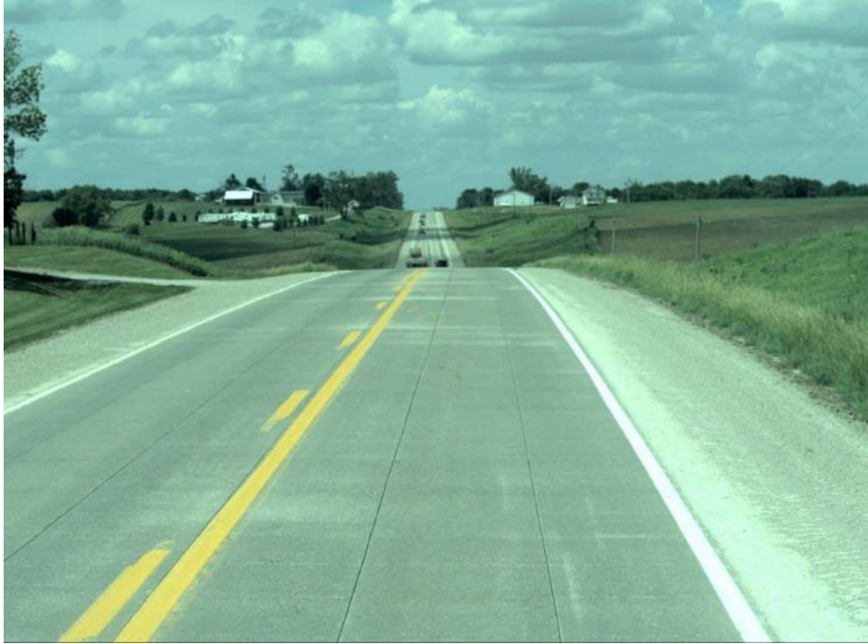
Figure 5 – 4-inch overlay 4 x 4 ft. Joint Spacing
