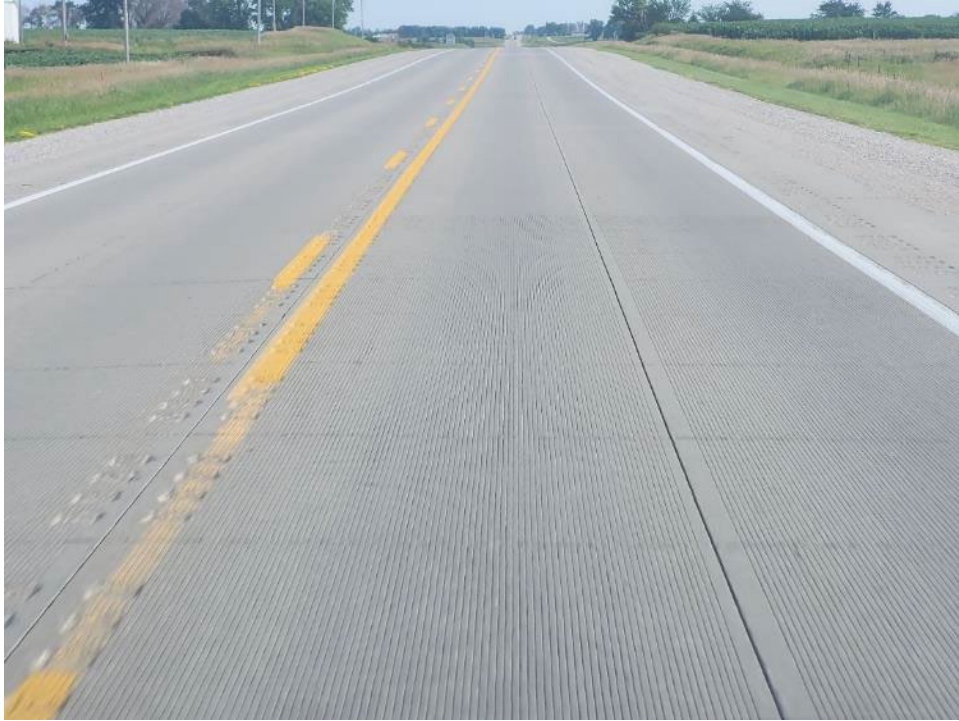
Figure 18 – Clay US 71 Whitetopping Built 2015
