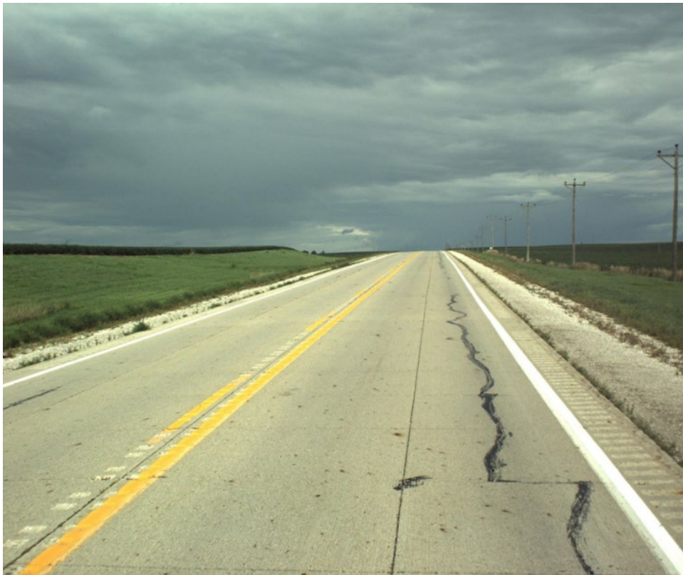
Figure 12 – Sac IA 175 UBOL Left Shoulder Crossslope 1.13%
