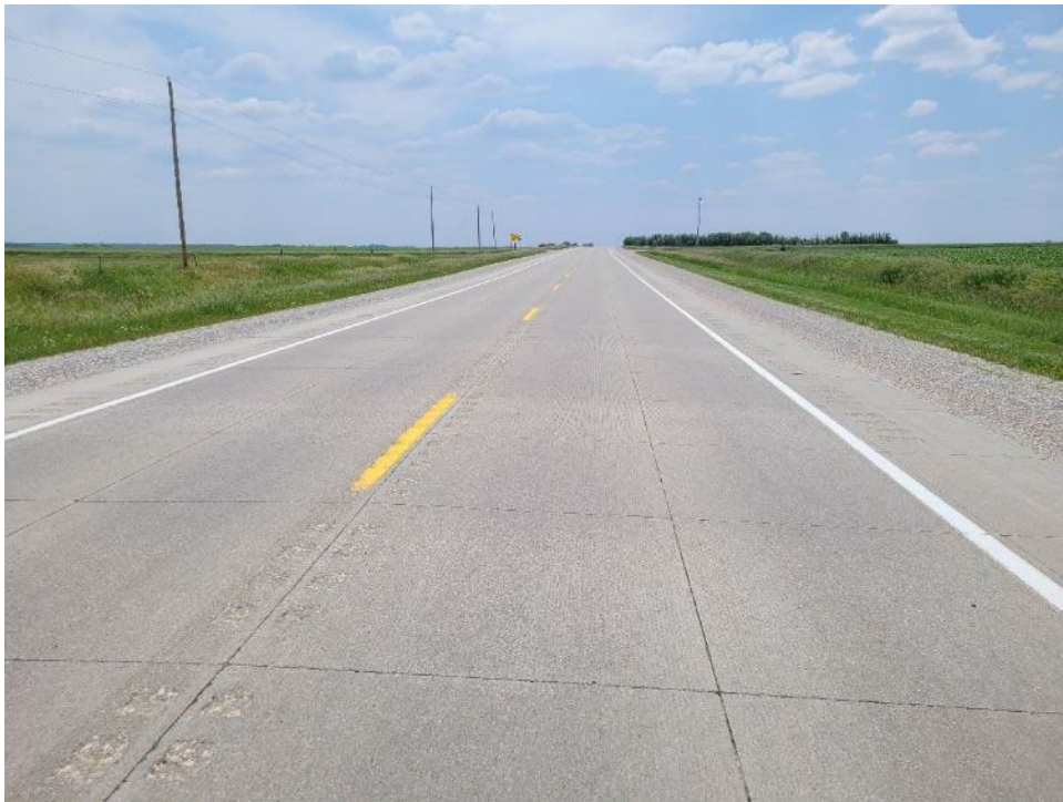
Figure 19 – Clay US 71 Whitetopping Built 2016
