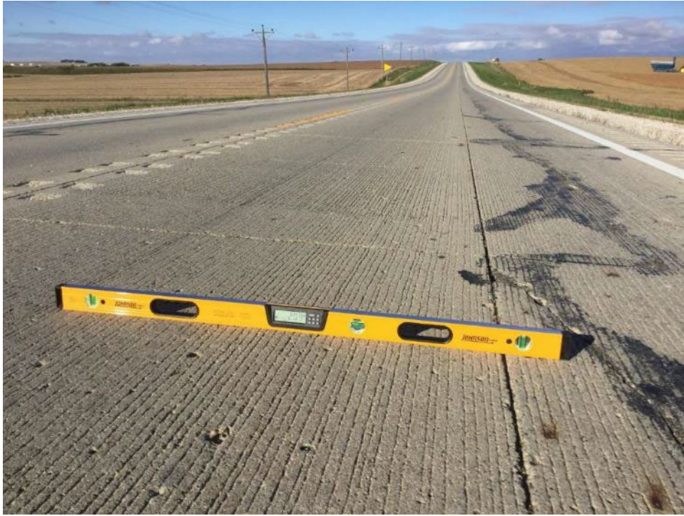
Driving lane panel cross slope 2.09%
