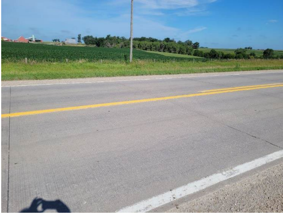
Figure 3 – 8-inch overlay 12 x 15 ft. Joint Spacing
