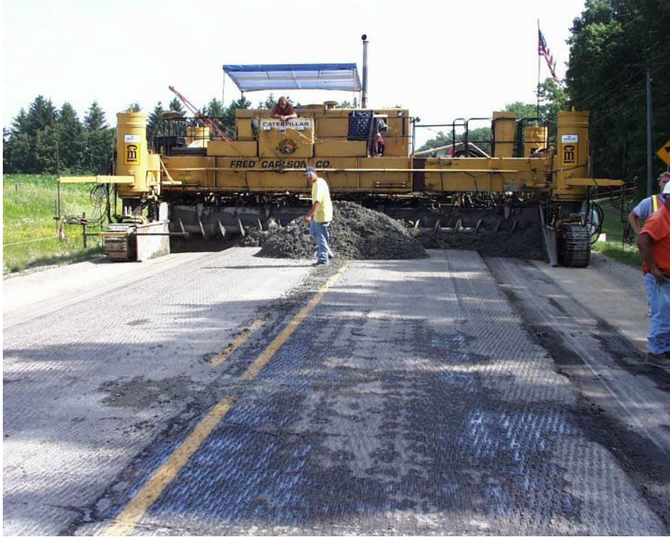
Figure 8 – Delaware IA 13 Unbonded Overlay Construction
