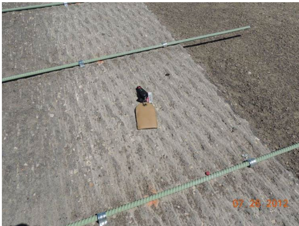
Figure 37 – Closeup of steel, stapled to existing pavement.
