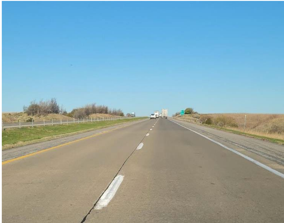
Figure 13 – Adair I-80 WB Whitetopping Overlay Paved 1979 (Picture 2023)
