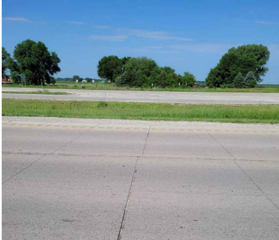
Figure 33 – Clay/Dickinson US 71 NB panels migrating in driving lane at BOP against HMA pavement.
