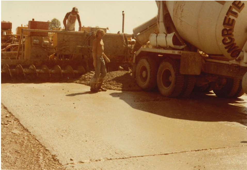
Figure 30 – Poweshiek I-80 Bonded Overlay 1984 with Grout on Existing Pavement
