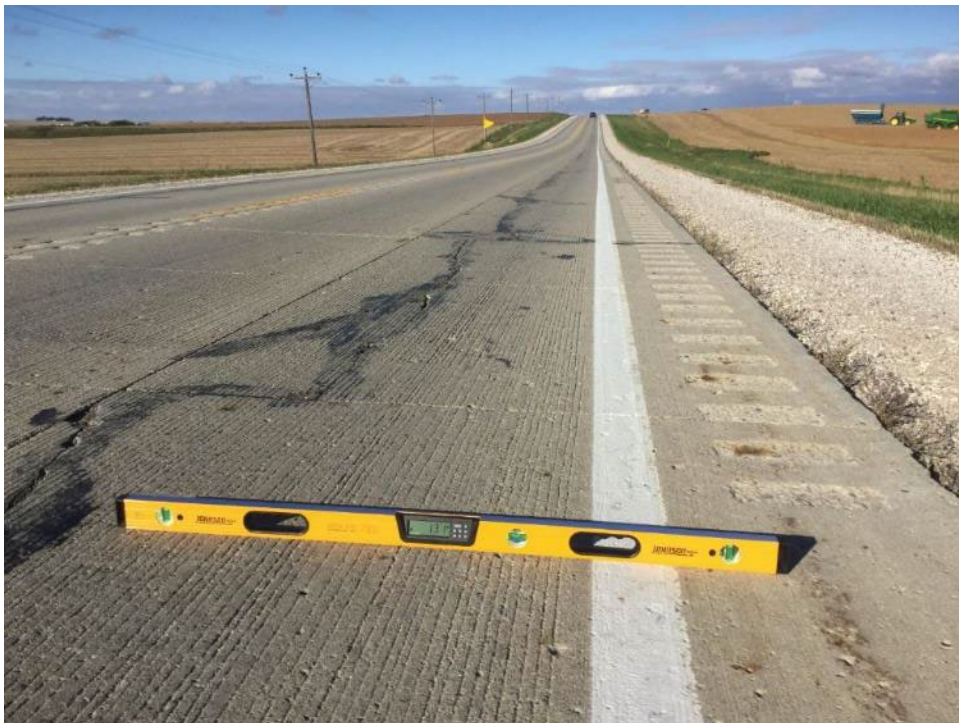
Shoulder panel cross slope 1.31%
