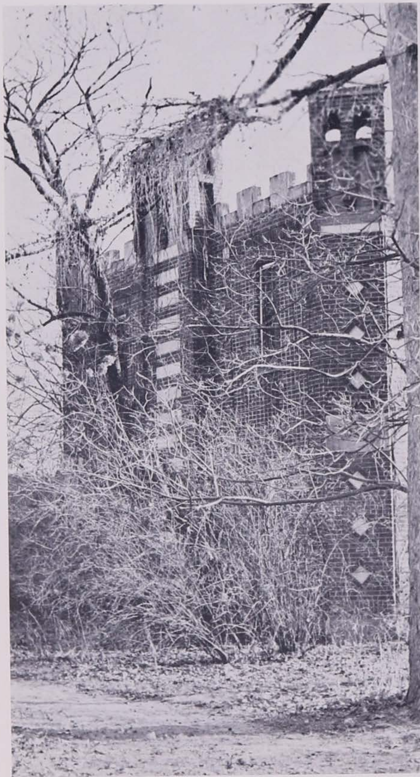
100 Ardenia (above and right), at 925 Kirkwood Avenue, is the exact opposite of the ideal of "honest" design so ponderously illustrated in the Courthouse. Its lowering, castle-like facade was added to an ordinary frame house. The wild and savage atmosphere of primitive warriors fighting meaningless battles with bows and arrows in the wilderness is greatly enhanced by the overgrown shrubbery and a decaying brick wall that surround it.
