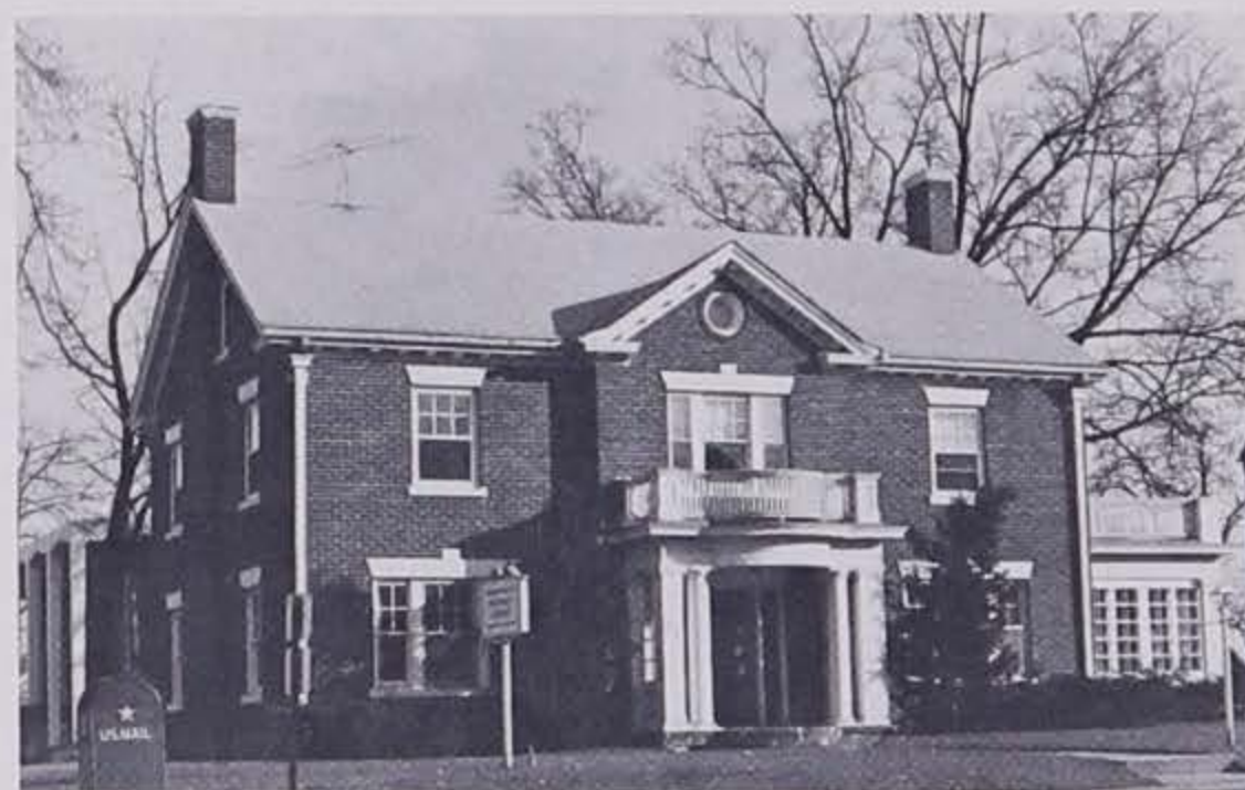
Oculi, the little round windows in gable ends, continued in vogue until the 1940s, demonstrating a remarkable continuity of taste. From the house at 829 Kirkwood Avenue, built in the 1870s; the College of Engineering at the southwest corner of Washington and South Capitol Streets, built in 1905; and the Baptist Student Center, at 230 North Clinton Street, built in the 1920s.
