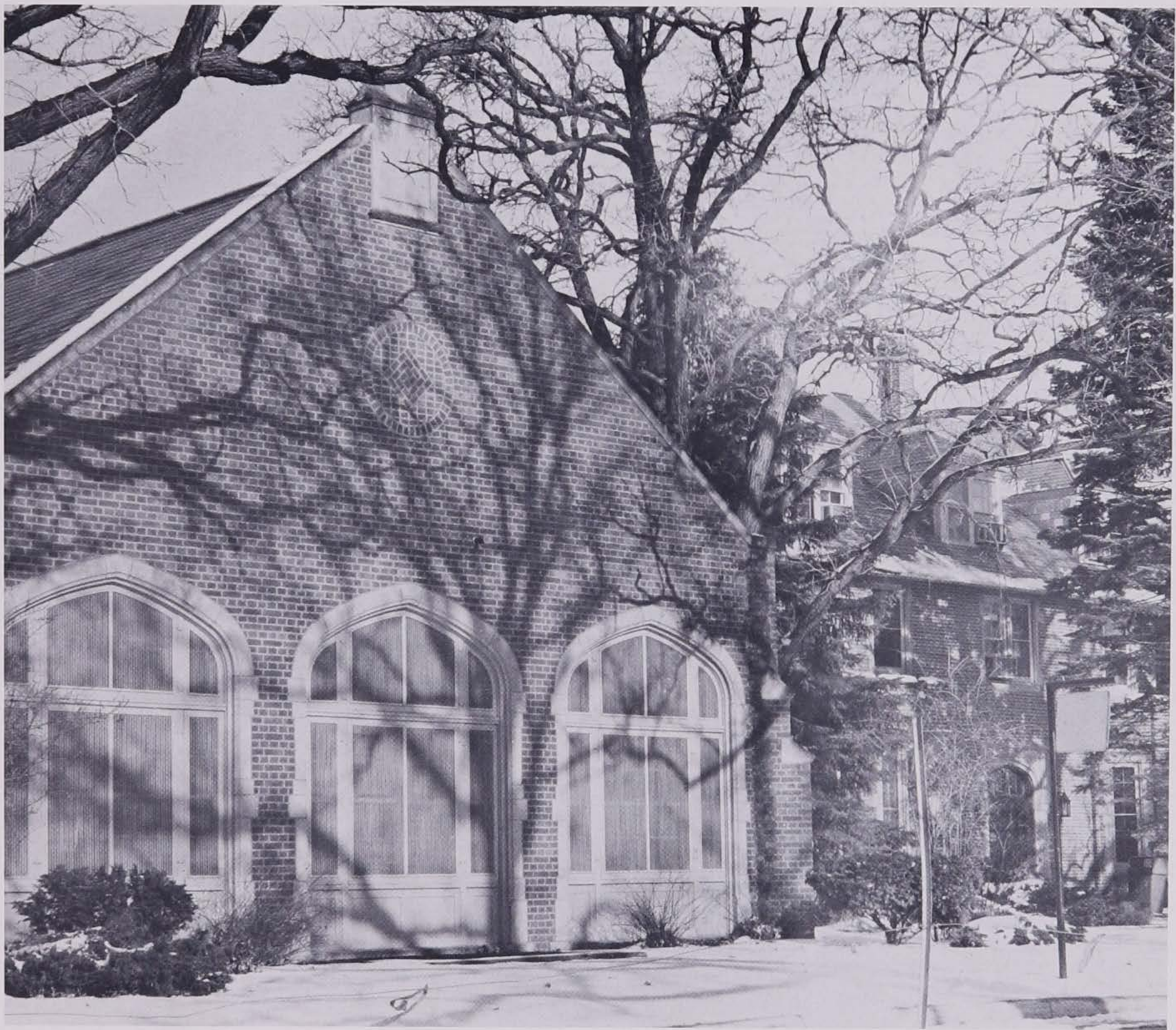
The University Psychopathic Hospital, on Newton Road was built in 1920. It reflects the Tudor (sixteenth-century English) sort of design popular at the time for schools, churches, hospitals, and shops. Casements, bay-windows, ornamental sandstone dressings, chimneys, steep-pitched roofs, little dormers, and construction in rose-colored brick, are all sufficiently authentic to mitigate the quite untypical expanse of blank wall and the rather slick, overtidy design.
