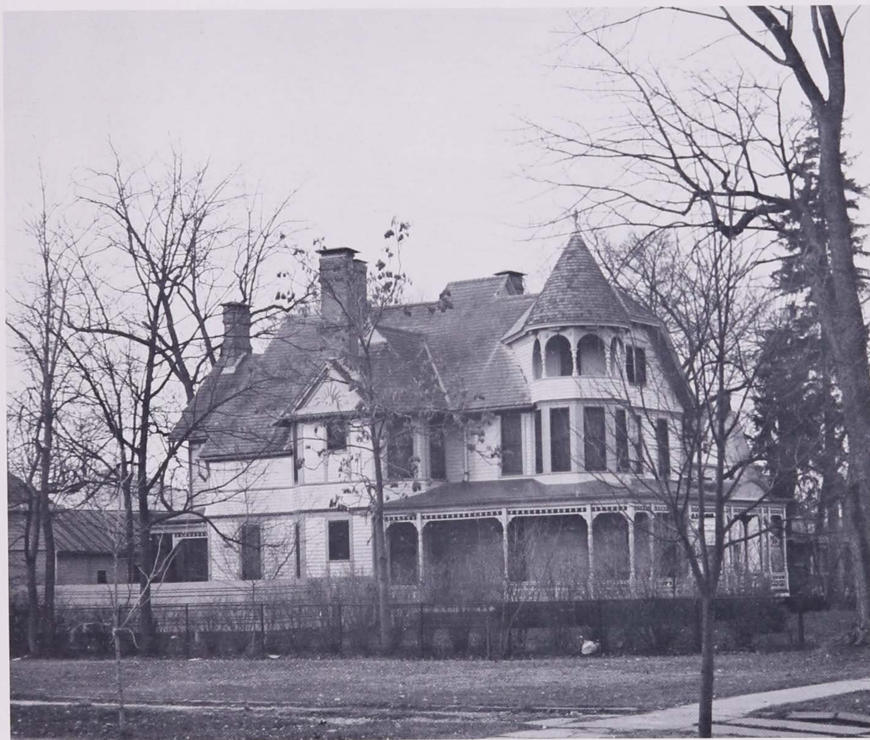
The Musser House, at 715 College Street, was built in 1890, at the height of the Queen Anne rage. It looks rambling, but this is an optical illusion; actually its fundamental plan is the simple, familiar Basic American, this time not a rectangle, cube, or L, but a cross. The tower is medieval in origin; the loggia was a staggeringly incongruous added amenity. The Musser House and another very like it at 1063 Woodlawn Avenue achieve dignity and a surprising atmosphere of tranquil comfort despite their varied and incompatible inspirations.
