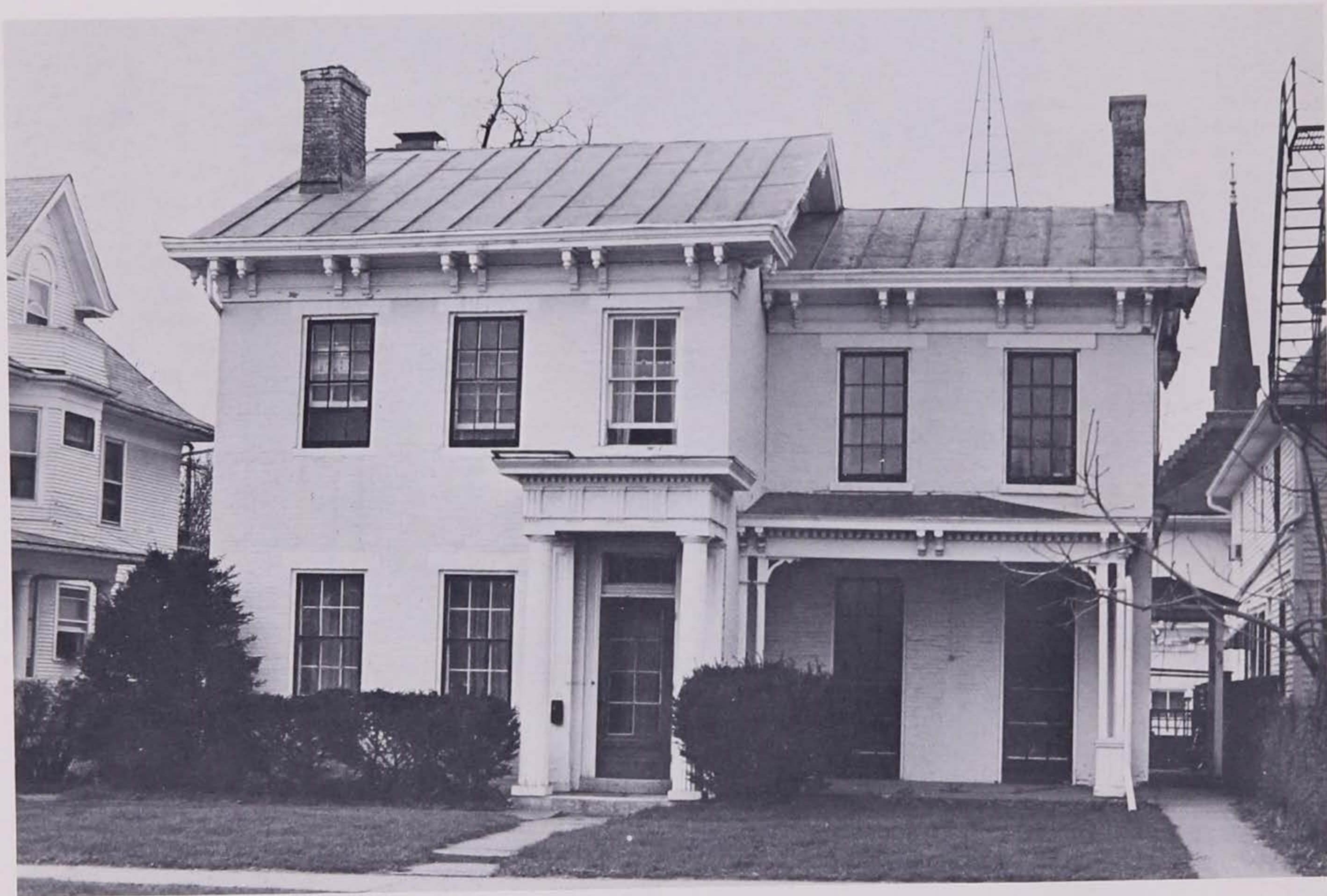
Page 6 President Gilmore's house at 109 East Market, from which the Doric column on p. 8 was taken, illustrates the way in which alien ornament began to be added to houses in the 1850s to dress them up. Under the paint that covers its brick, the Gilmore House is very similar to Plum Grove, but it is a little
