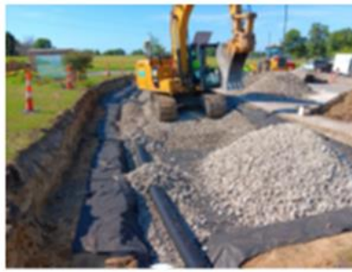
Figure 2: Placing storage aggregate for pavers.
