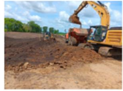
Figure 3: Excavation of the wetland at Mustang Lane.
