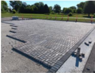
Figure 1: Permeable pavers in place at Fross Park
