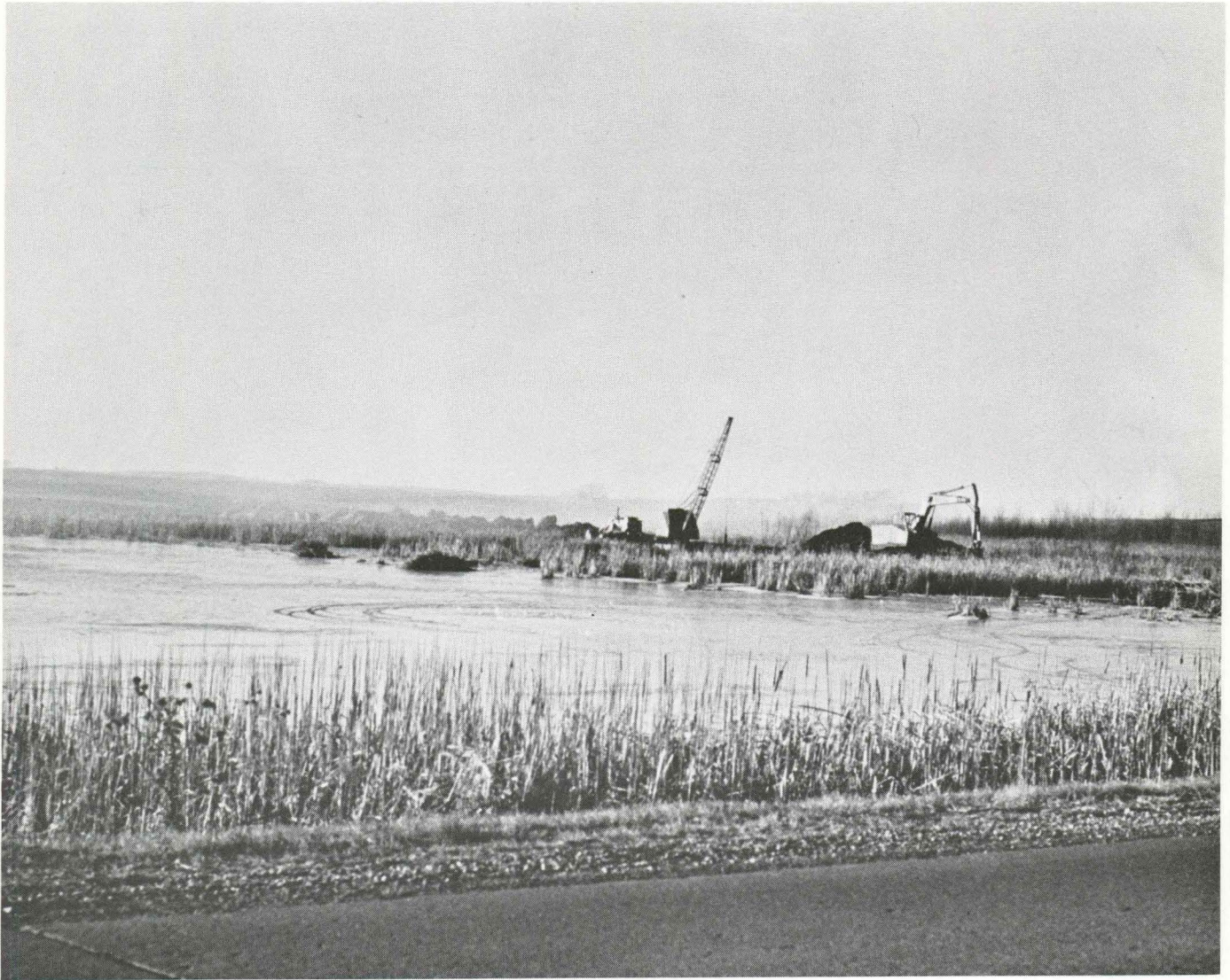
Fig. 2. Prairie marsh being drained by construction of drainage ditch.
