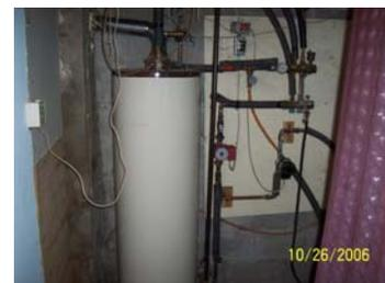
*This is a picture of a water heater that the client had rigged to heat the building. The water heater used pipes under the floor to radiantly heat the house. The problem is that when they take a shower, all the hot water is expended and there is not hot water to heat the house.*
