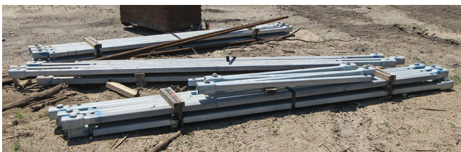
Figure 3. Helical pile extension sections
