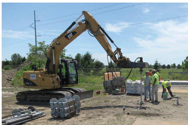
Figure 4. Helical pile installation equipment
