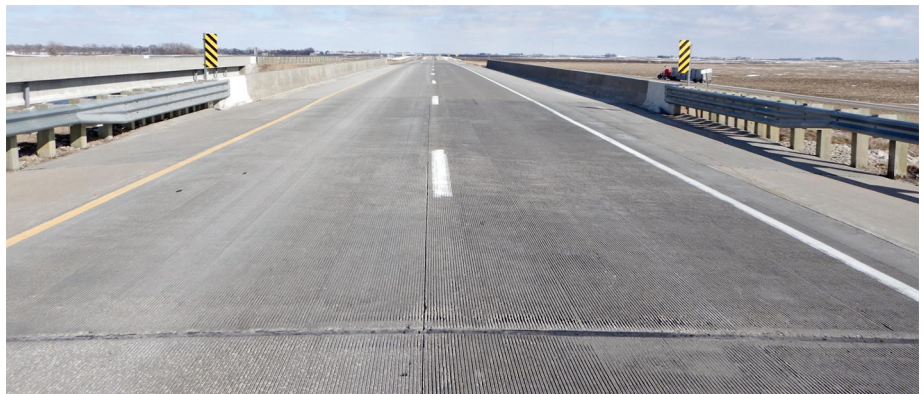
Integral abutment bridge and approach slab
