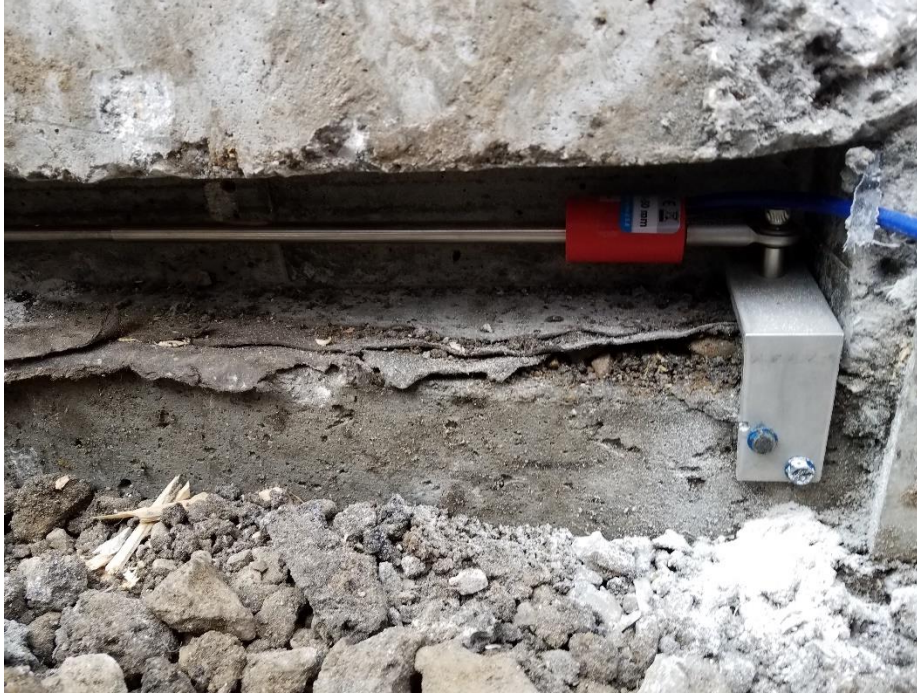
Figure 4.28. Story County 118—crackmeter approach slab side blackout location
