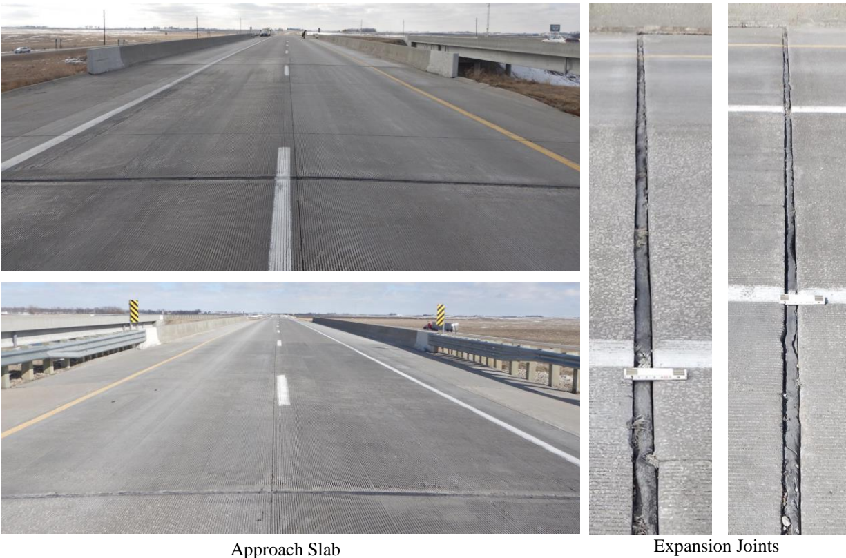
Figure 2.40. Bridge inspection photographs—approach slabs
