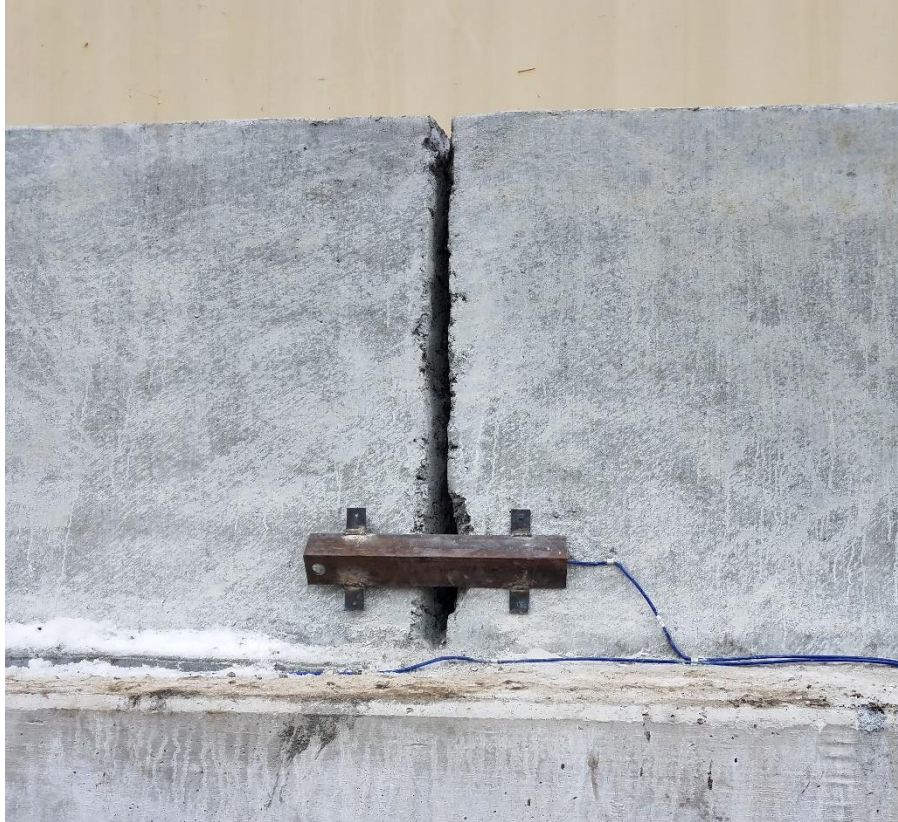
Figure 4.27. Story County 118—crackmeter installation across the barrier rail joint
