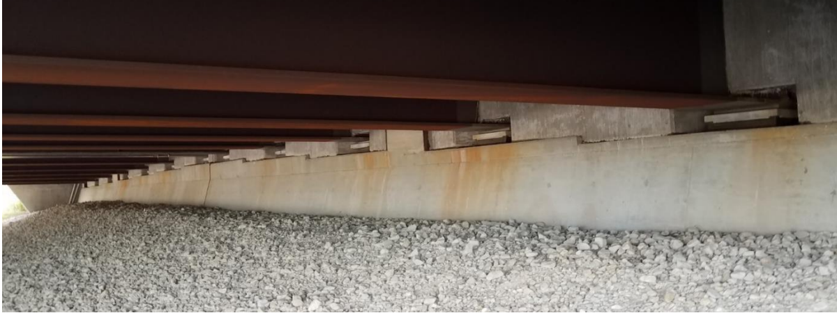
Figure 3.2. North abutment face
