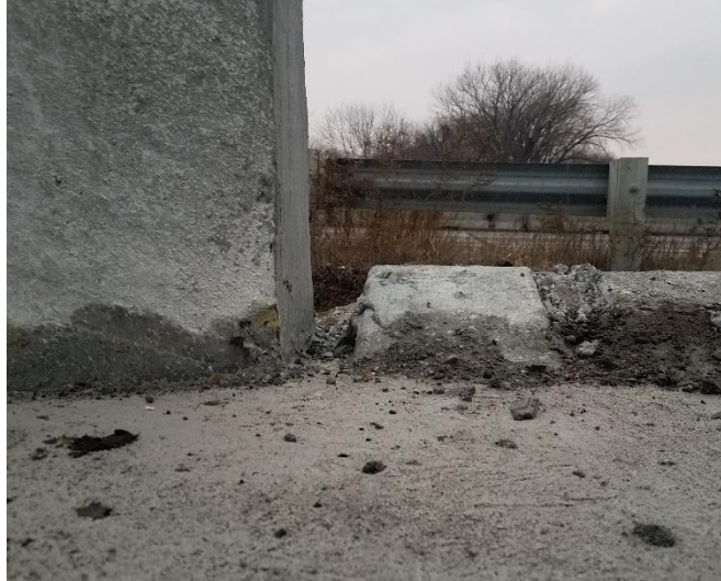
Figure 4.40. Story County 118—curb gap at the barrier end (typical)
