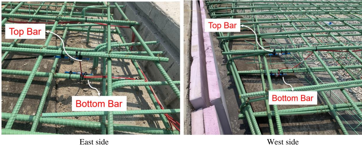
Figure 4.64. Butler County 118—strain gauges installed on the longitudinal rebar
