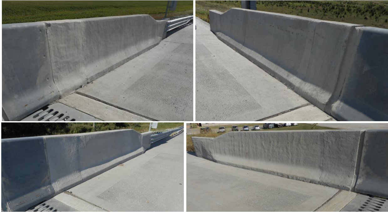
Figure 2.47. Bridge inspection photographs
