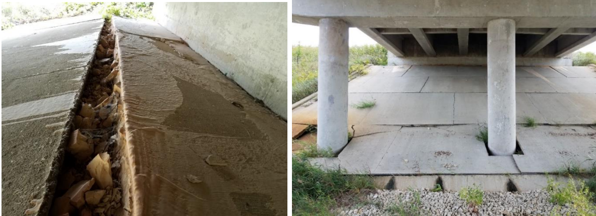
Figure 3.11. Typical embankment condition (left) and embankment condition at the abutment (right)
