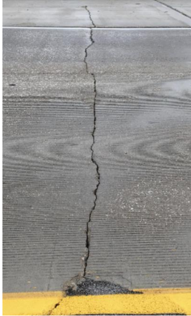
Figure 2.31. Transverse cracking
