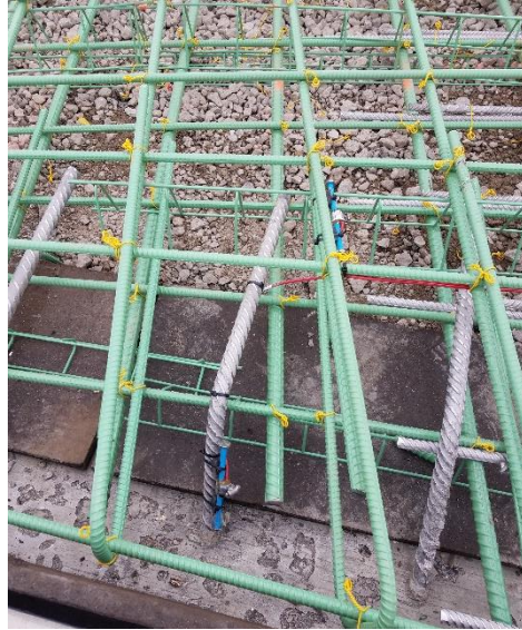
Figure 4.43. Story County 118—approach slab modified subbase condition immediately before concrete pouring
