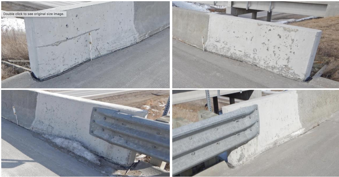
Figure 2.41. Bridge inspection photographs—barriers
