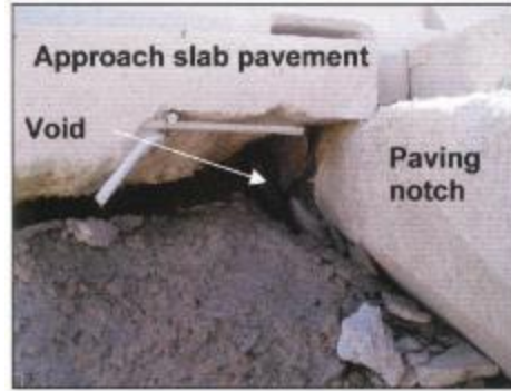
Figure 2.22. Voiding under approach slab
