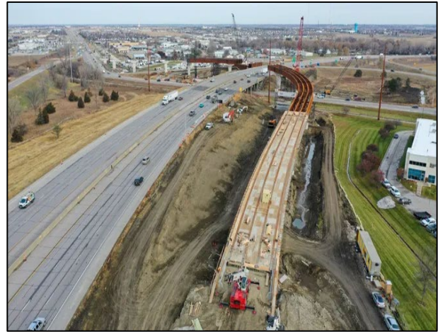
Figure 2. Hwy 141 Flyover at I-35/I-80 – Urbandale (circa 2023)
