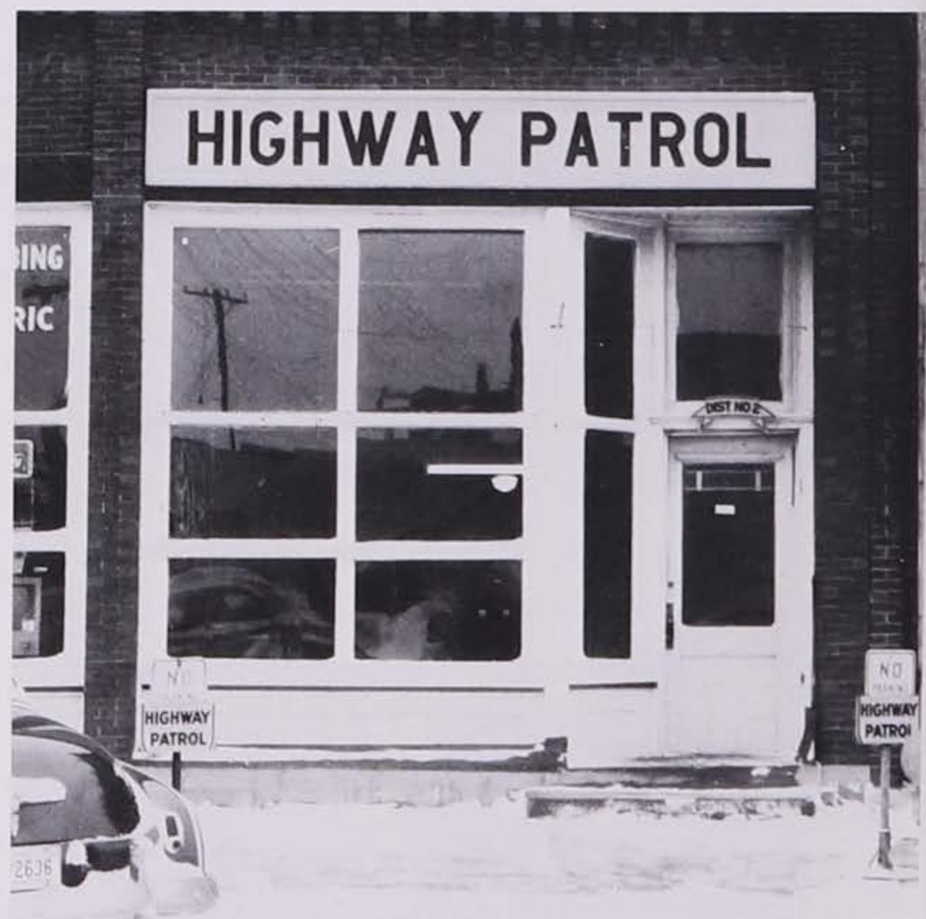
District 2 office on the south side Osceola town square.
