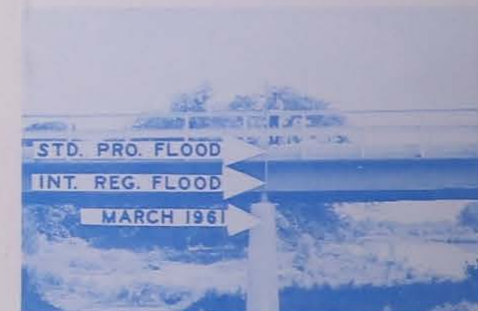
Upstream side of county Road "Z" Bridge
