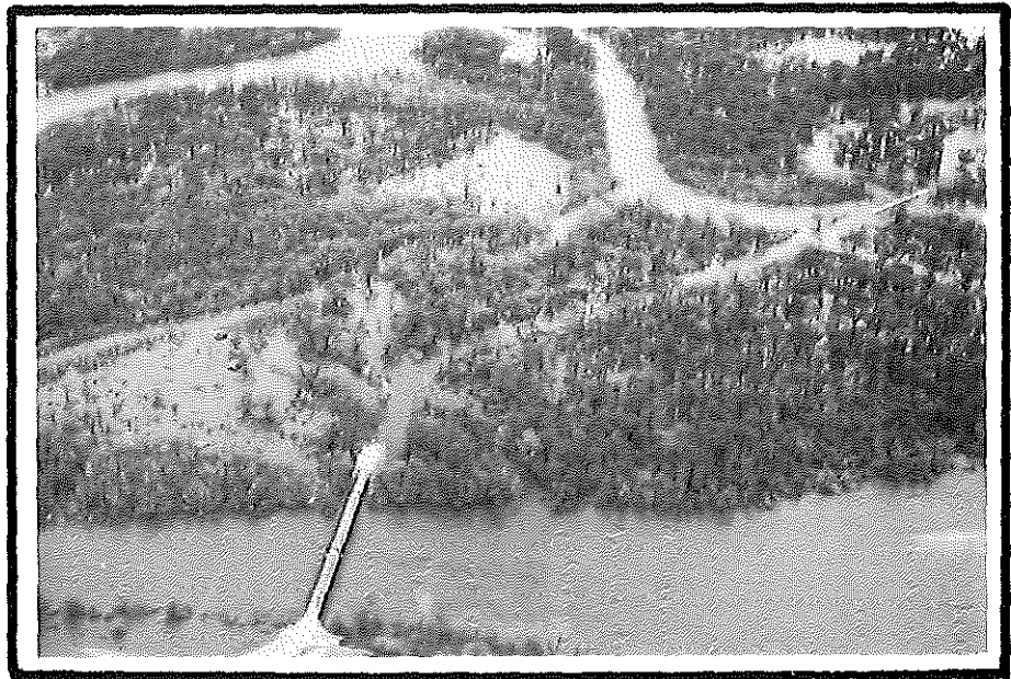
Figure 15. FLOOD SCENES - 31 March 1961. Top view is looking downstream at the C.R.I. and P. R.R. bridge at Mile 126.56 and the C.M.St.P. and P. R.R. bridge at Mile 126.44. Bottom view is the County Road bridge near Palo at Mile 129.74. Note the submerged approaches to the bridges and flooded overbank areas.
