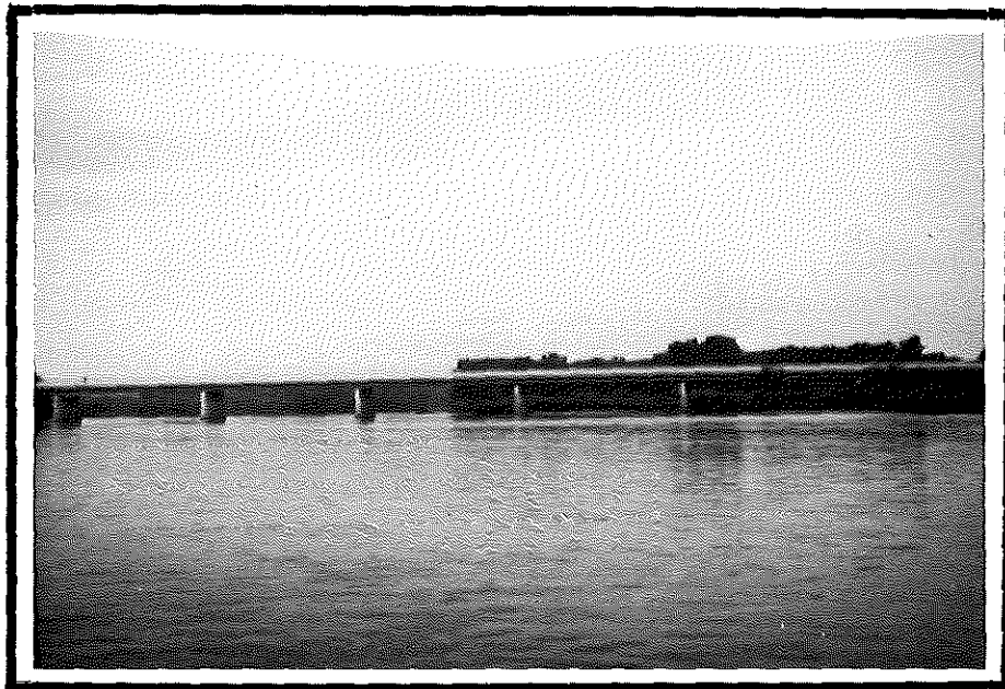
Figure 11. CEDAR RIVER BRIDGES AND DAMS Top view is looking upstream toward the County Road bridge near Palo at Mile 129.74. Bottom view is the County Road Z bridge at Mile 138.90, looking upstream.
