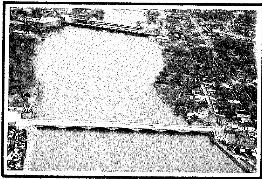
Figure 12. FLOOD SCENES - 31 March 1961. Bottom view is looking upstream with 16th Avenue bridge in the foreground. Top view is looking upstream with the C.M.St.P. and P. R.R. bridge and 8th Avenue bridge in the foreground and city government buildings on the island in the center of the photo.
