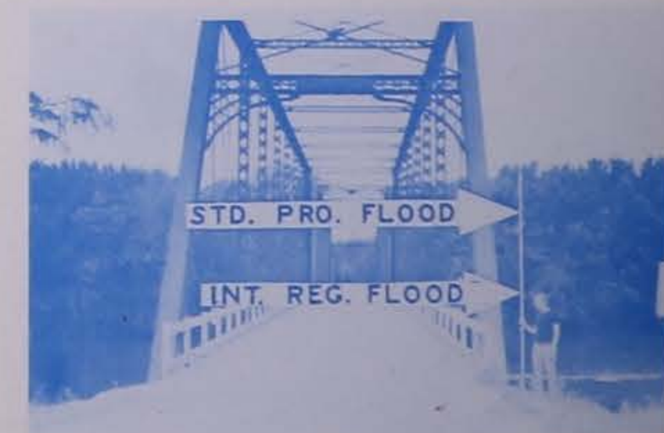
Right bank of Chain of Lakes Bridge near Palo
