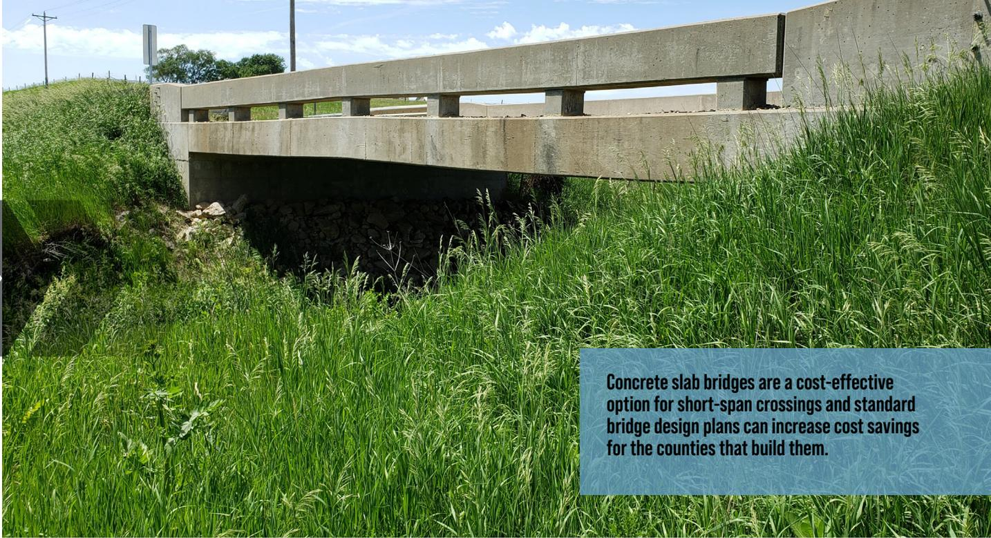
Concrete slab bridges are a cost-effective option for short-span crossings and standard bridge design plans can increase cost savings for the counties that build them.
