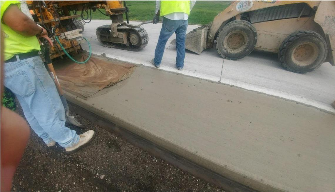
**Figure 6: Paving with PEM Shoulder Mix**
