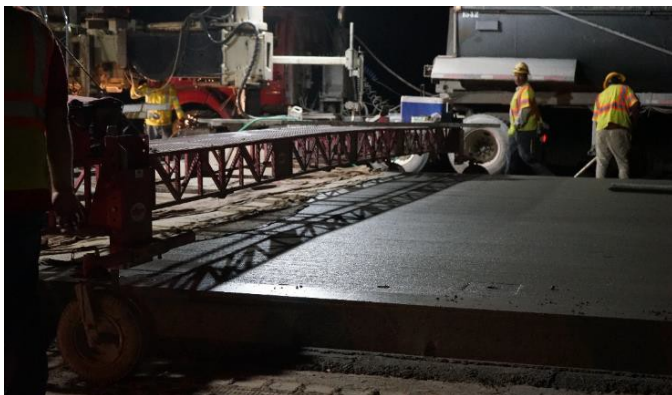
Finish and Edge of the pavement immediately after being constructed.
