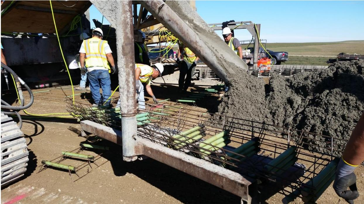
The base was reworked on the project and gravel pre-trimmed, but left a little high. The “Iowa Special” unloading machine also performs the final trim of the base course cushion material leaving a fresh uniform cross section and base for the new concrete surfacing.
