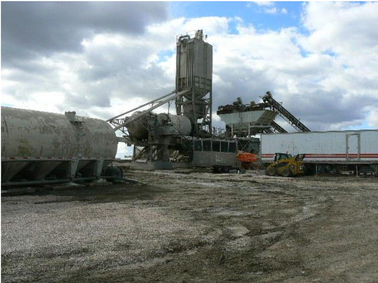
Weather became a factor during the paving operations. October and November in South Dakota that year were wet and cold at times. Equipment and plant break downs also delayed paving operations. Reede was able to place from 2,000 ft to 3,500 ft per day of the 26' wide 10.5" PCCP on full production days. On these days, the plant would produce from 1800 to 3200 yd<sup>3</sup> per day.
