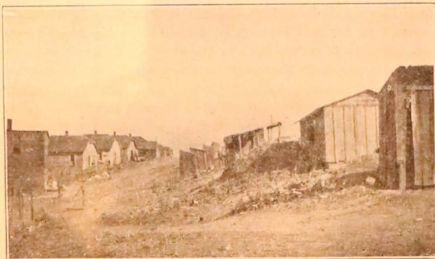
Such conditions should not exist in Iowa. Note manure rubbish, row privies and well at foot of slope below privies.
