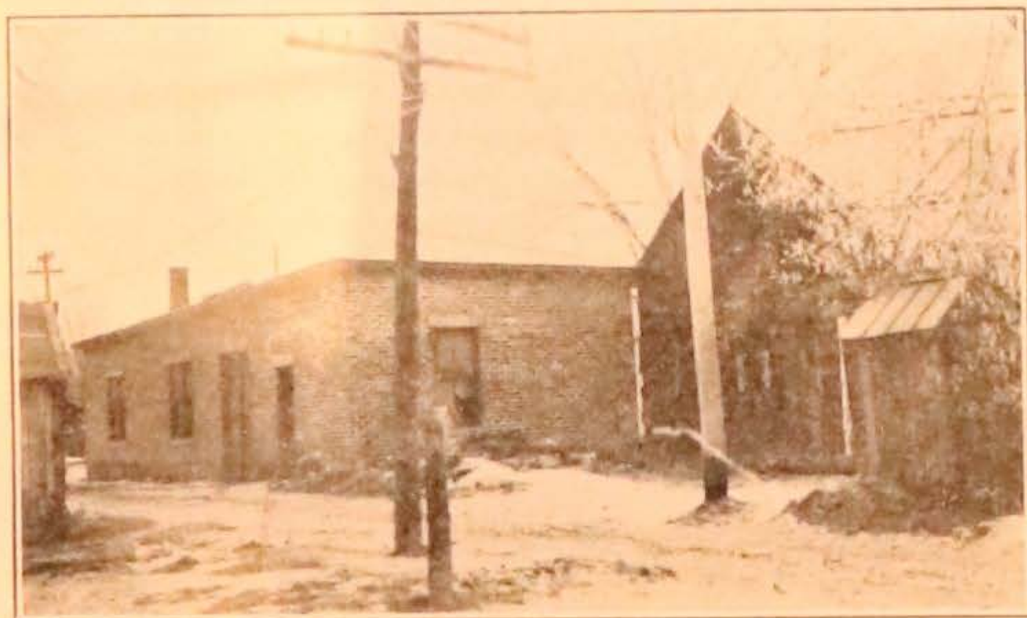
A poorly located city well. Note privies at right and left within few feet of well. Well is under brick building.
