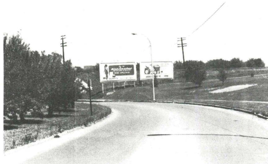
No Delineators or Pavement Markings to Define Curve or Approaching Underpass
