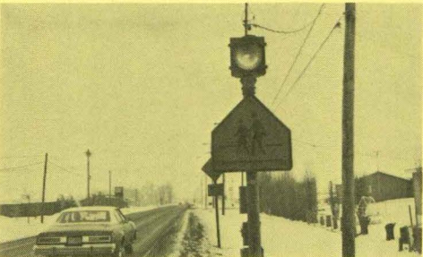
G Assembly on E 1st St., 30" Type S2-1 (incorrect usage) should be Sign A assembly. Flashing beacon is on continuously--incorrect usage.
