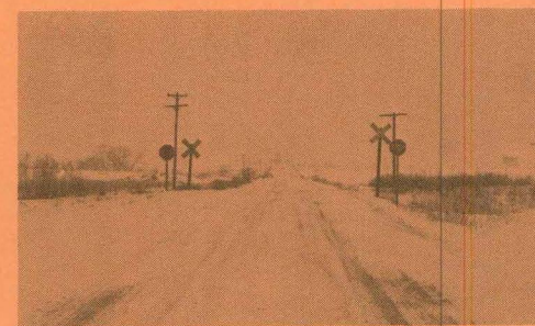
L 102nd STREET--East of NW 16th St.--Looking West
