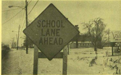
E Nonstandard sign on W 1st St.--should be 36" Type S1-1.
