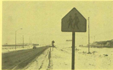
B 36" Type S1-1 Advance School sign for use on approaches to school areas.
