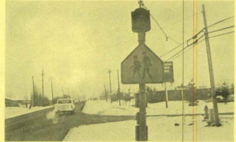
F Assembly on E 1st St., 30" Type S1-1 sign should be 36" size and add panel as in Sign A. Yellow flasher operates correctly--morning, noon, afternoon periods.
