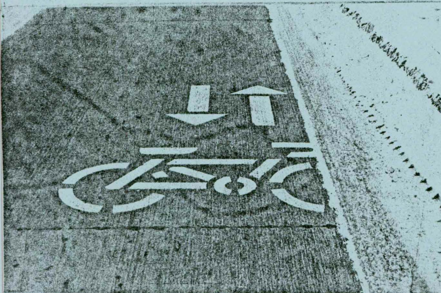
Nonstandard symbol marking, approximately 125 in place along designated routes.
