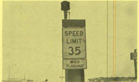
I Assembly on N Ankeny Blvd. Operates on SchoolDays 7-9am, 11am-1pm and 3-5pm.
