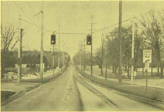
A Typical span-wire supported school crossing signal on a two-lane arterial, approximately 75 feet from intersection.
