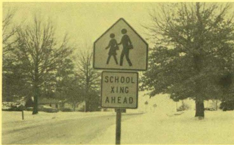
A Assembly recommended for approaches to designated school crossings--36" S1-1 sign and 24" panel.
