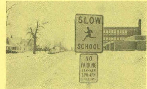
H Nonstandard sign near Junior-High--Should be 36" Type S1-1 (Sign B).
