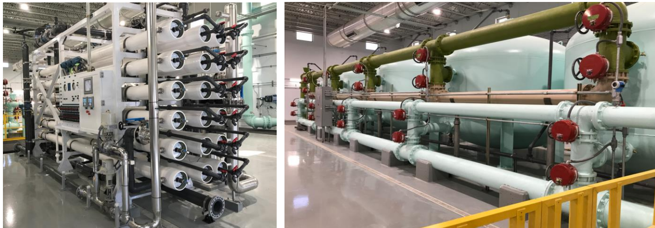
New water treatment plant constructed primarily in 2021.
