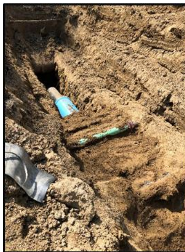
Water main installation using open trench construction (photos were provided by the system)
