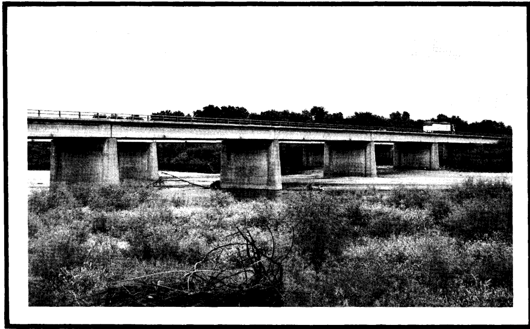
Figure 9. Looking northeast at the downstream side of the eastbound lane of Interstate 80 & 35 twin bridges - Mile 209.10.
