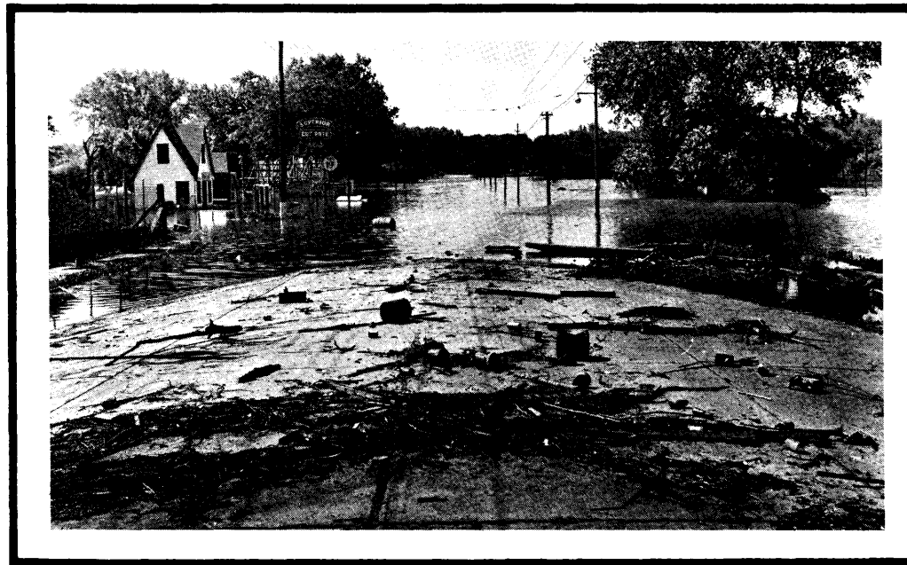
Figure 20. Looking south on Sixth Avenue from New York Avenue - Mile 204.28, during the flood of June 1947.
