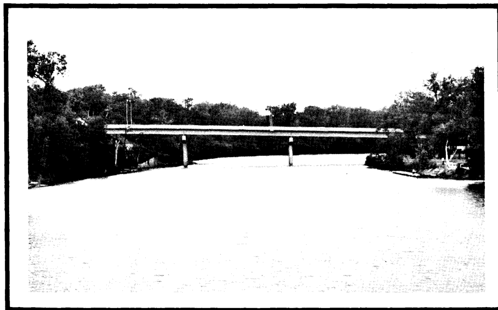
Figure 6. Looking upstream at the Sixth Avenue bridge - Mile 204.58.
