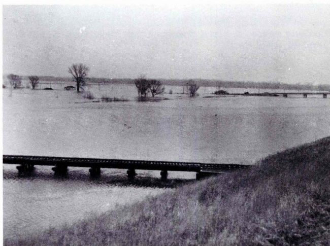
Looking northeast at the D.M. & C.I. R.R. and Beaver road bridges over Beaver Creek — April 10, 1965 flood.
