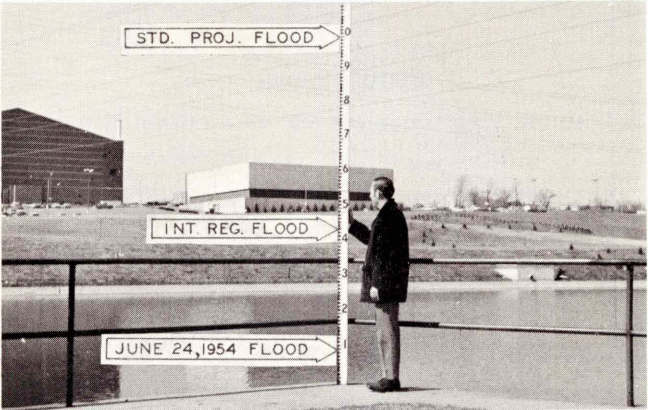
North walk on the left end of Center Street dam.
