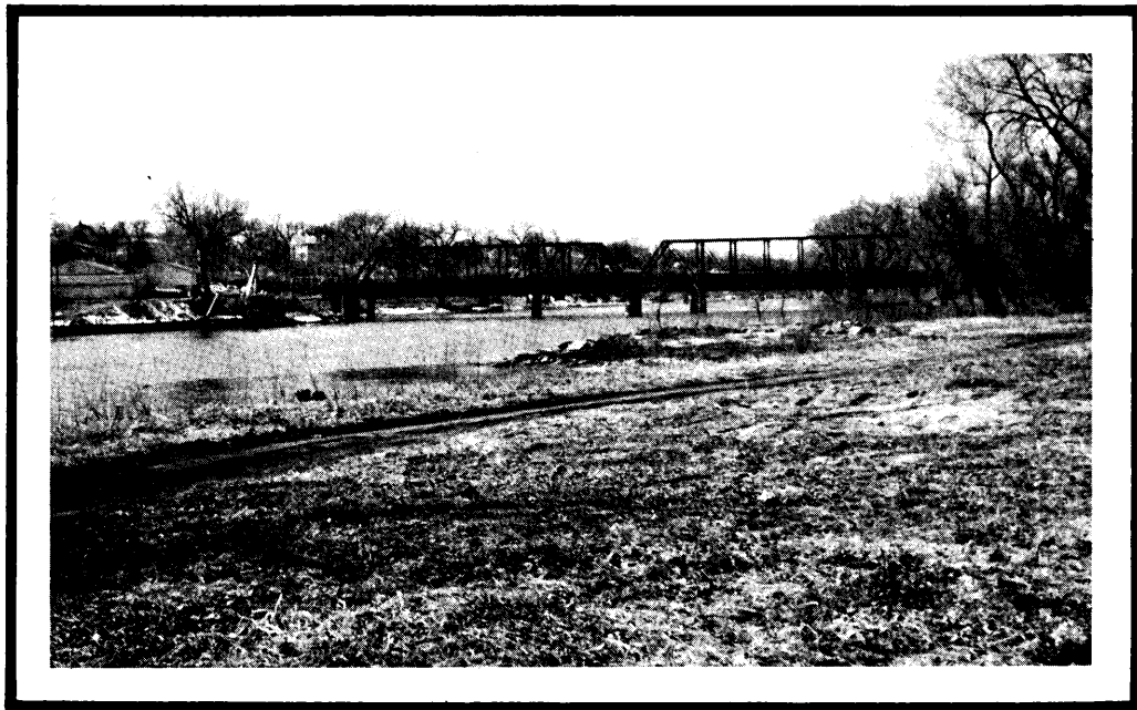
Figure 4. Looking upstream at the D.M.&C.I. RR bridge - Mile 204.28.
