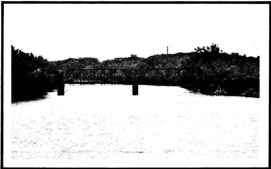
Figure 7. Looking downstream at the D.M.&C.I. RR bridge - Mile 206.10.
