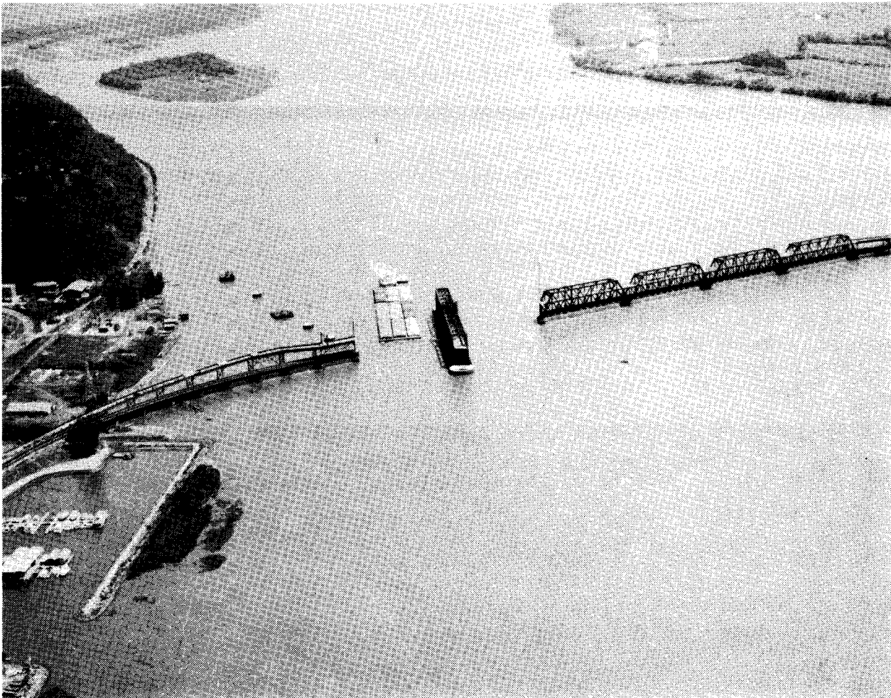
Swing Span Bridge in Open Position, Fort Madison, Iowa
