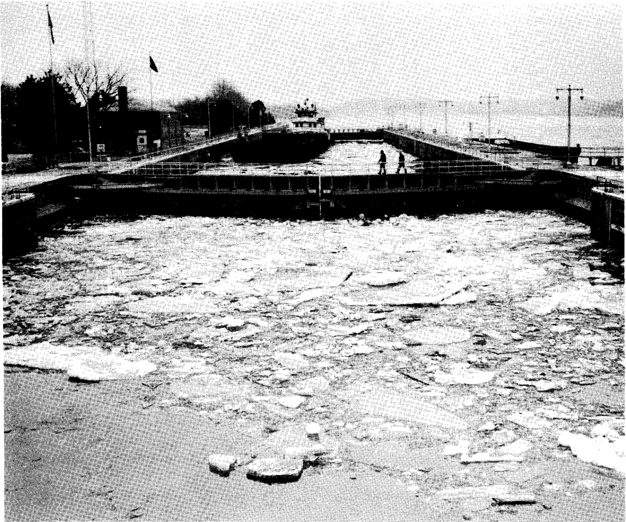
Locking Through Under Icy Conditions, Lock 16 Photo - Courtesy of Corps of Engineers
