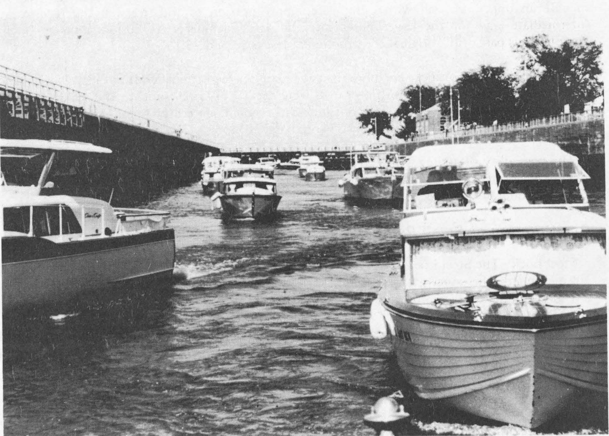
Recreational Craft Leaving Lock Chamber, Lock & Dam II, Dubuque, Iowa
