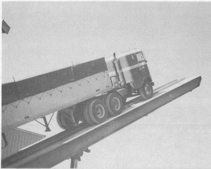
Truck Hoist at Mississippi River Grain Terminal
