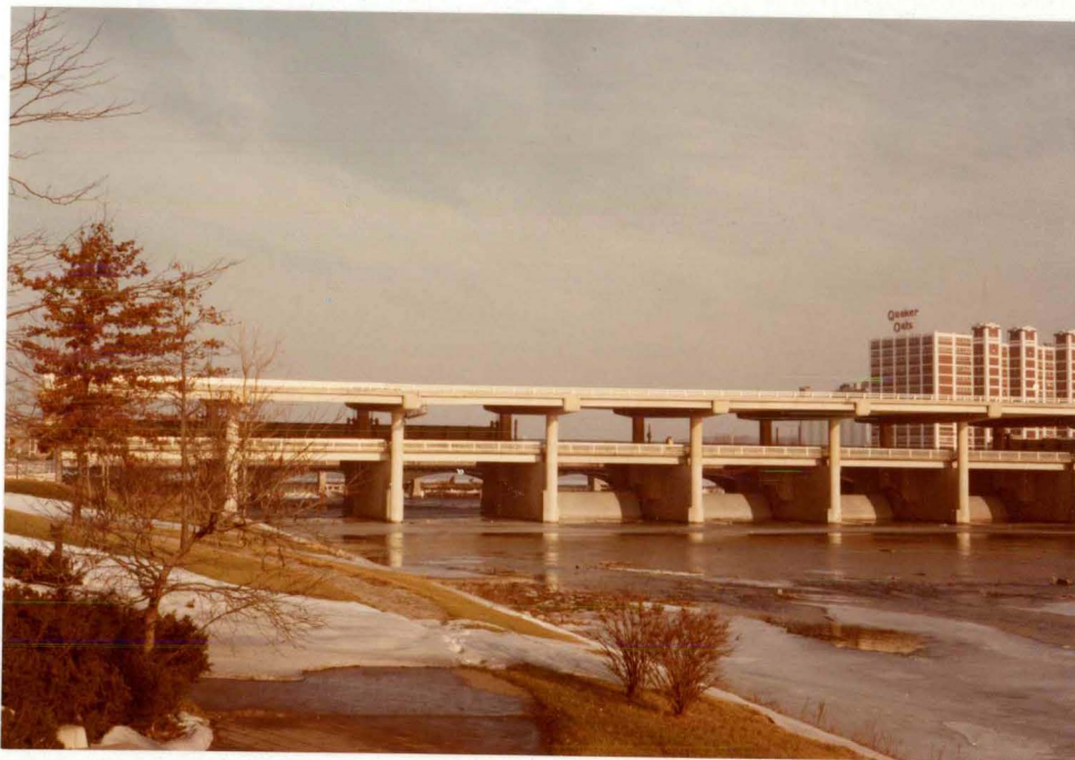
View of the structure looking northeast from the west bank city park development.
