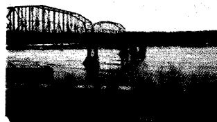
VIEW OF BRIDGE STRUCTURE
