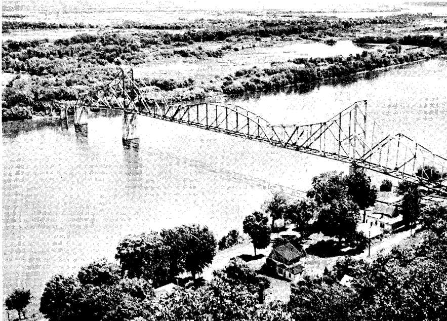
IOWA SIDE OR WEST CHANNEL CROSSING
