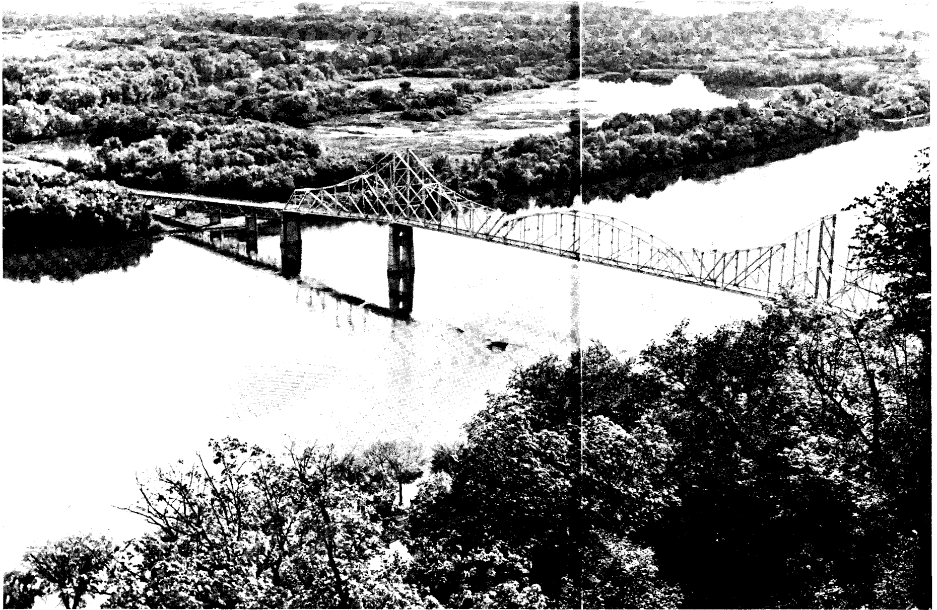
VIEW OF BLACK HAWK BRIDGE FROM LANSING, IOWA LOOKING SOUTHEAST
