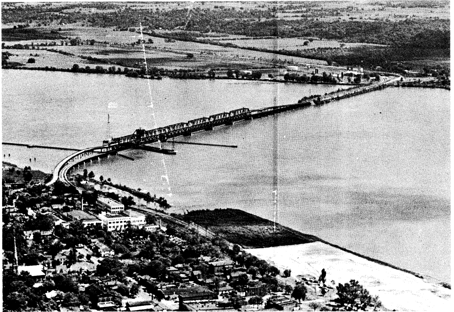
VIEW OF A.T.&S.F.R.R. BRIDGE FROM FORT MADISON, IOWA, LOOKING SOUTHEAST
