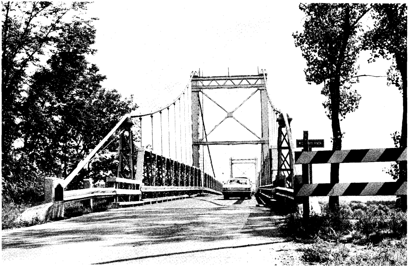
Exhibit I-2 EXISTING MAIN CHANNEL SPAN PRAIRIE DU CHIEN BRIDGE
