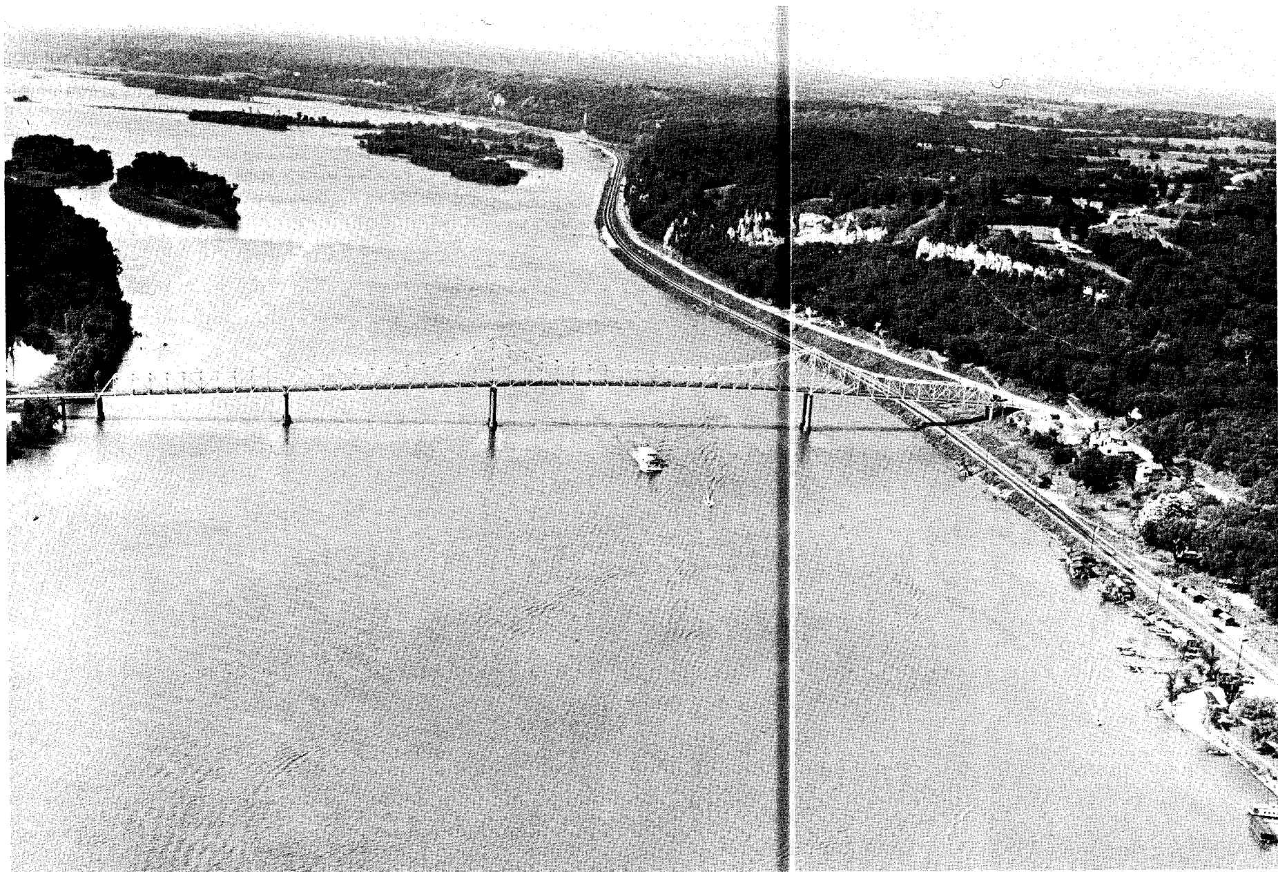
VIEW OF SAVANNA-SABULA BRIDGE LOOKING NORTHWEST
