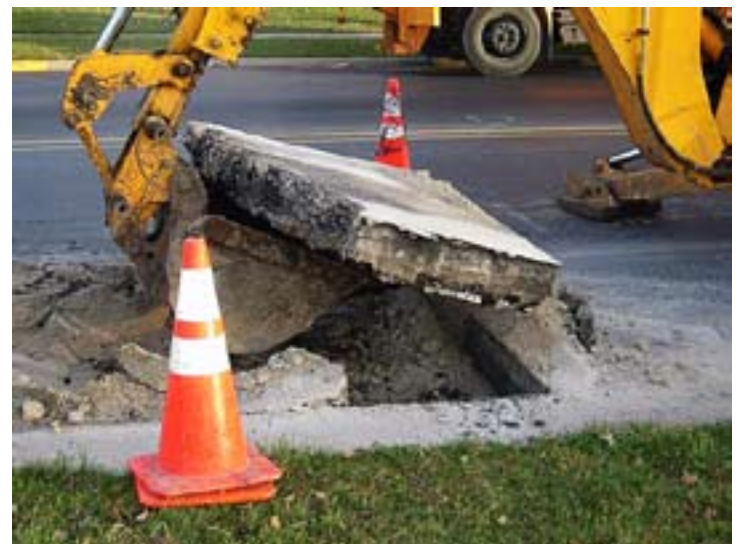
Pavement removal
