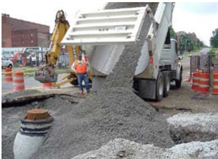
Large backfill lift being placed
