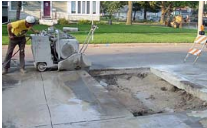
Concrete pavement cut being made
