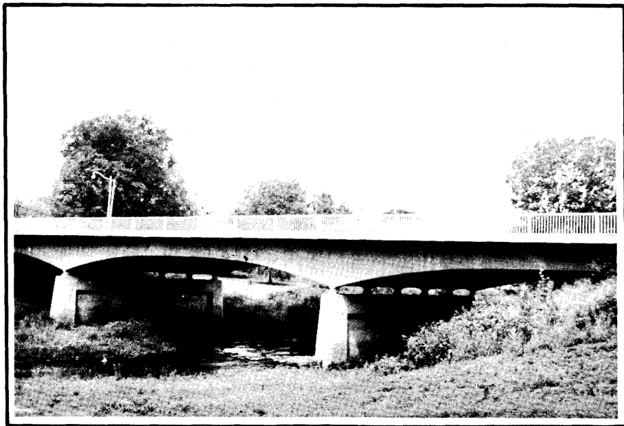
Marion Boulevard Bridge Mile 10.81. Looking Upstream at Bridge which carries Highway 151, 64 and 94 traffic.
