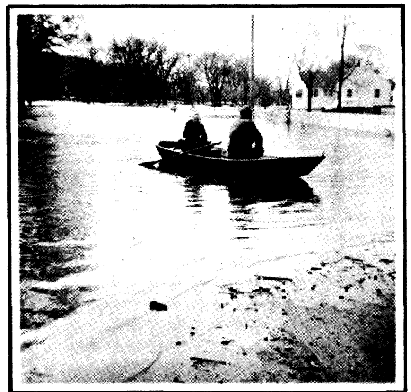
Photo 5 - Boating on County Road "GG" looking south toward the Indian Creek main channel during the March 1961 Flood at Mile 0.75.
