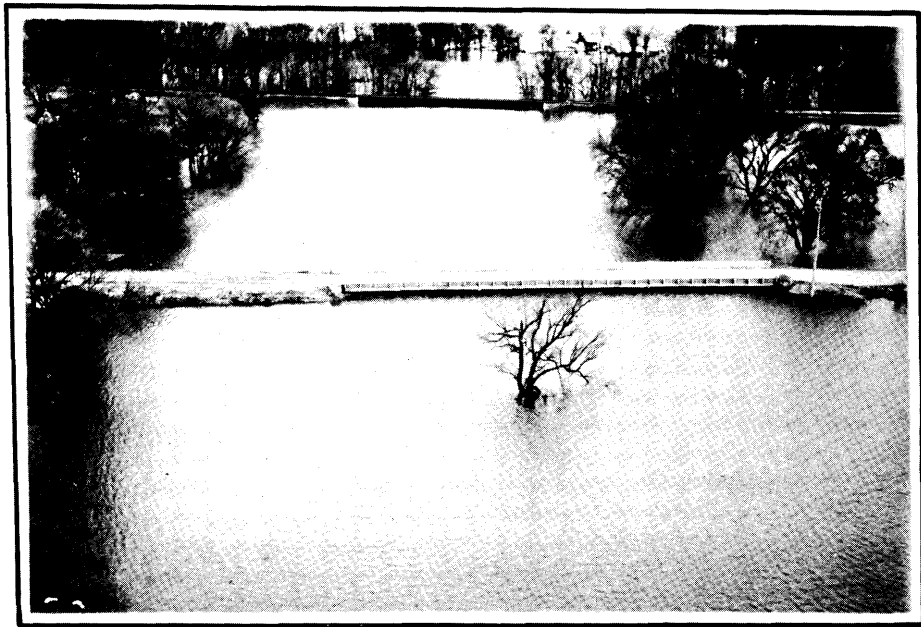
Photo 3 - Otis Road Bridge in foreground and C. & N.W. Railroad bridge in background during the April 1960 flood. Looking downstream at Mile 0.18.
