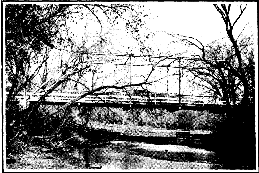
County Road Bridge Mile 2.21. Looking Downstream at Bridge and cattle guard.
