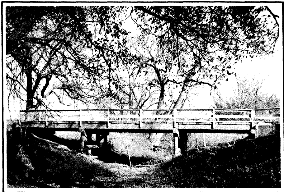
Council Street Bridge Mile 15.10. Looking Downstream from the center of Dry Creek.
