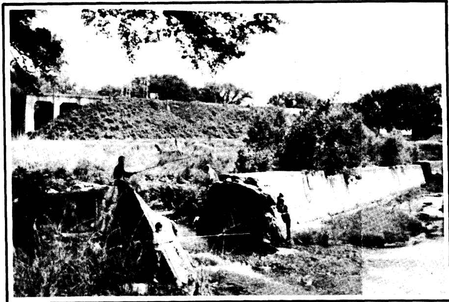
Old East Star Mill Dam Mile 10.90. Looking Upstream at toe of dam showing profile of removed section.
