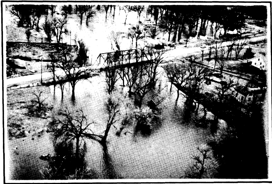
Photo 1 - Mt. Vernon Road Bridge during the April 1960 Flood. Looking downstream at Mile 1.08.
