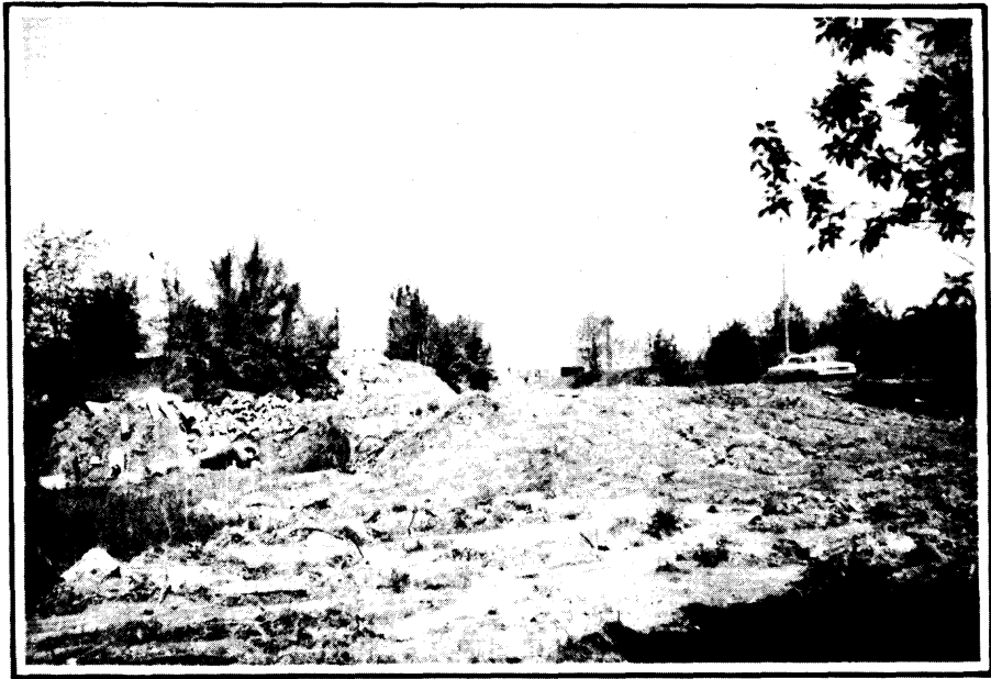
Photo 14 - Filling on Indian Creek flood plain at end of 40th Street Drive S.E. projected. Photo taken from right bank of Indian Creek located in Cedar Rapids, adjacent to Marion-Cedar Rapids Corporate City limits at Mile 7.80.
