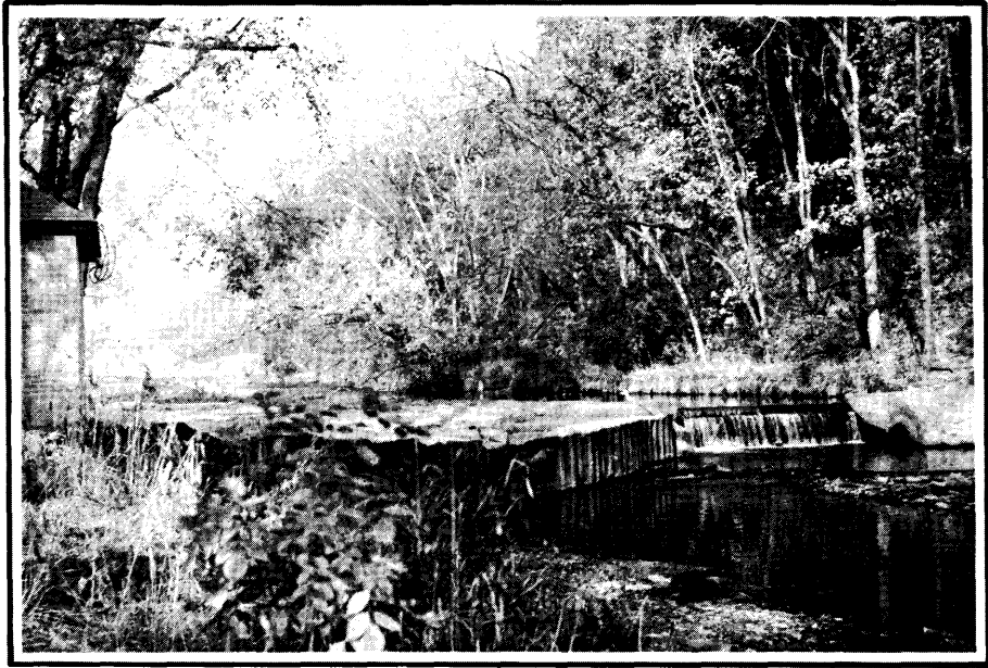
Cedar Rapids Country Club Dam Mile 6.20. Looking Upstream at Dam and Pump House for Sprinkler System.
