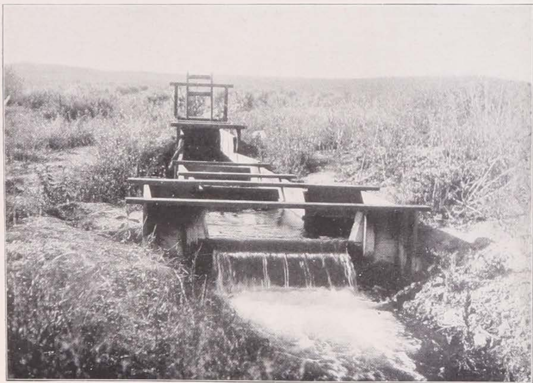
FIG. 2.—A CIPPOLETTI MEASURING WEIR.
