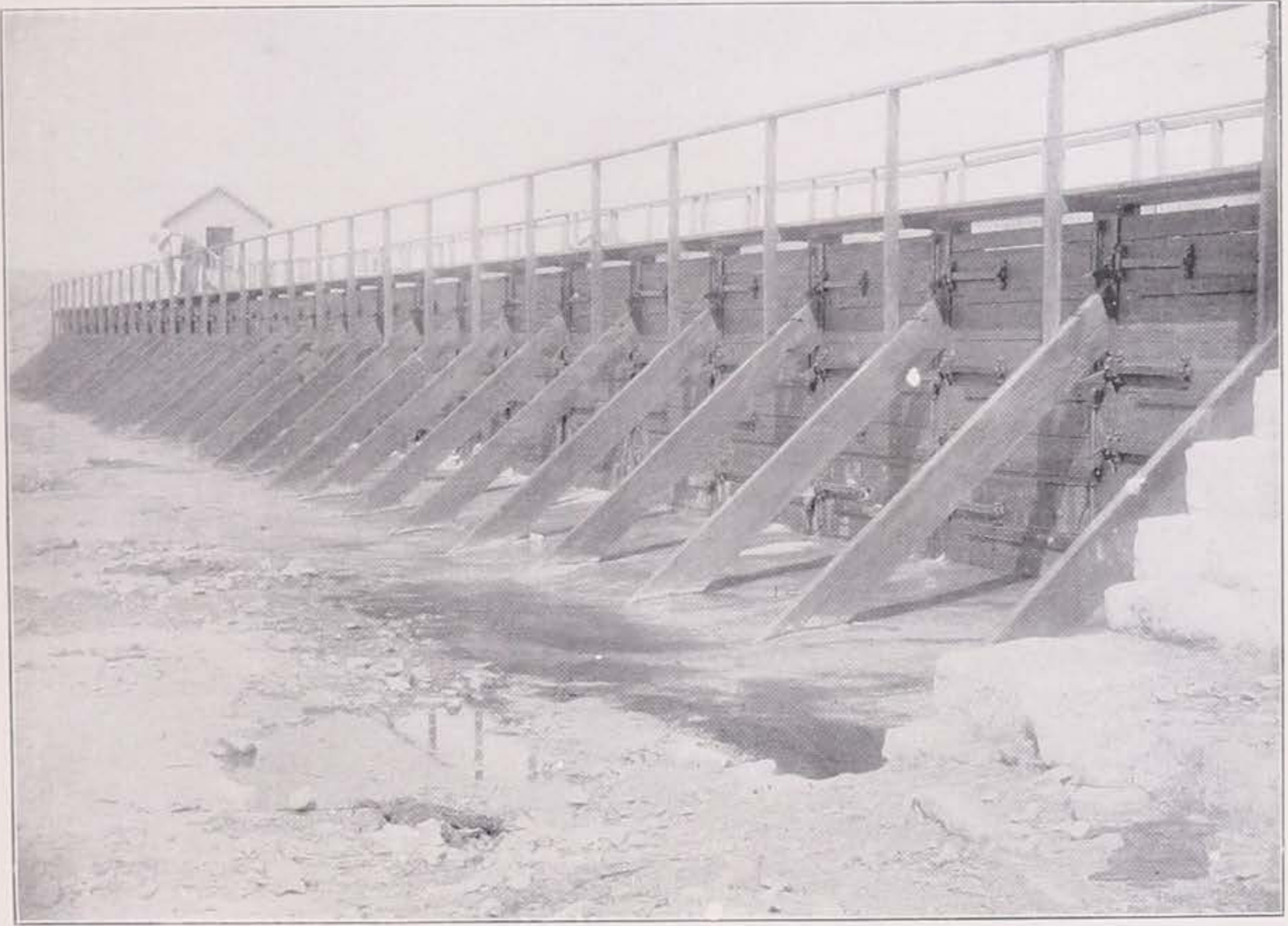
FIG. 1.—CANAL WASTE GATE CLOSED.
