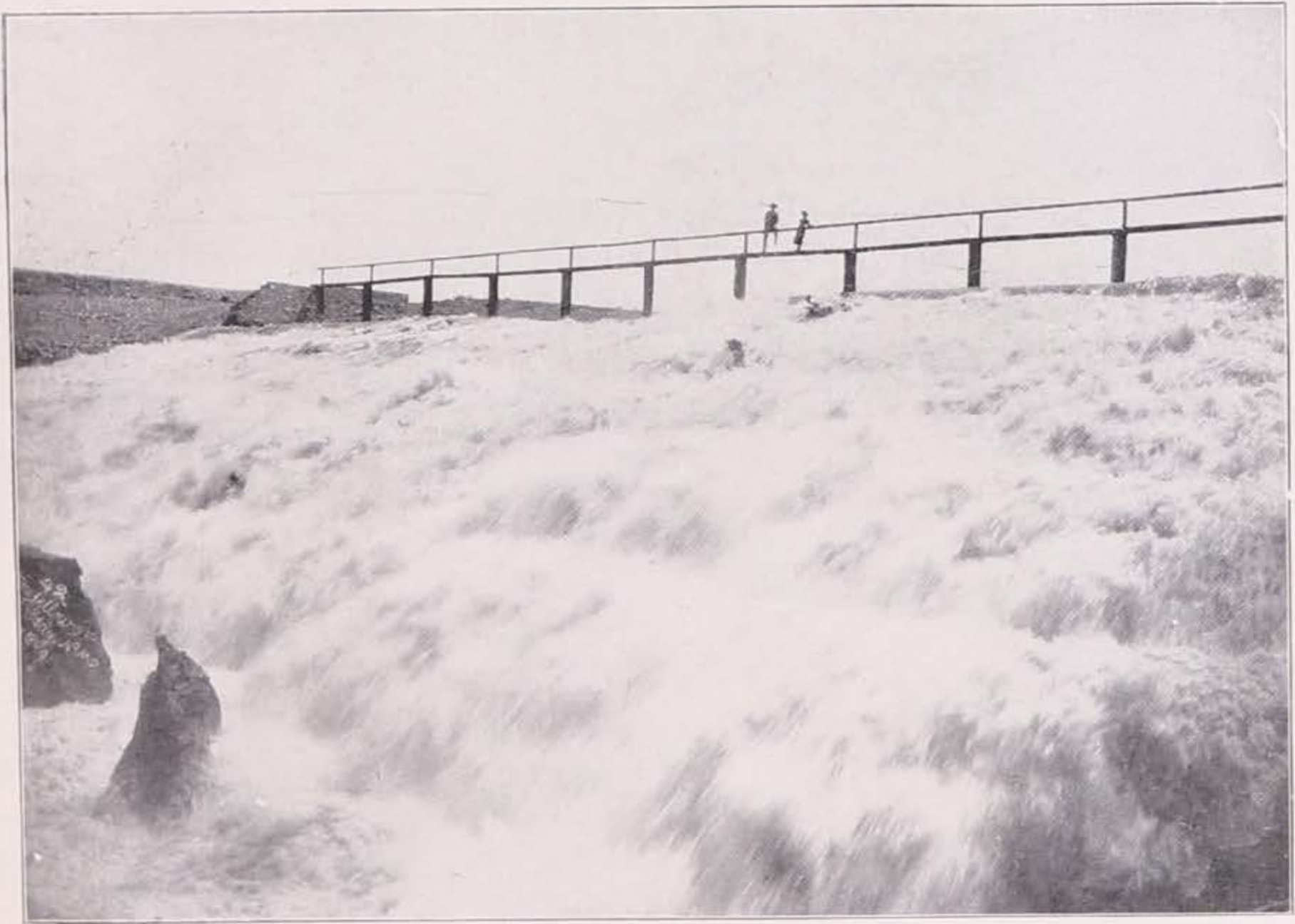
FIG. 2.—CANAL WASTE GATE OPEN.
