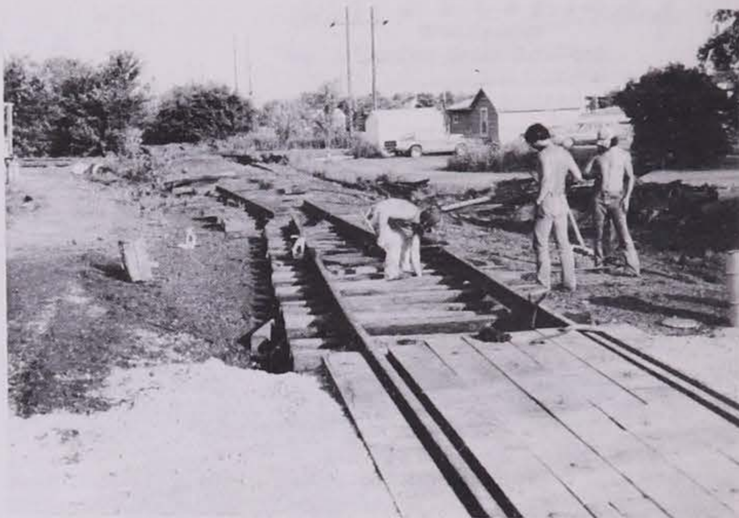
Kewash rebuilds track. Connection to Milwaukee Railroad. N. Ave D. August, 1983
