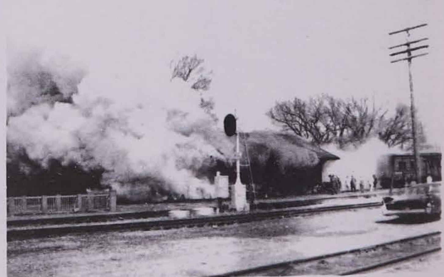
Milwaukee Freight Depot. Continues to Burn. April, 1964.
