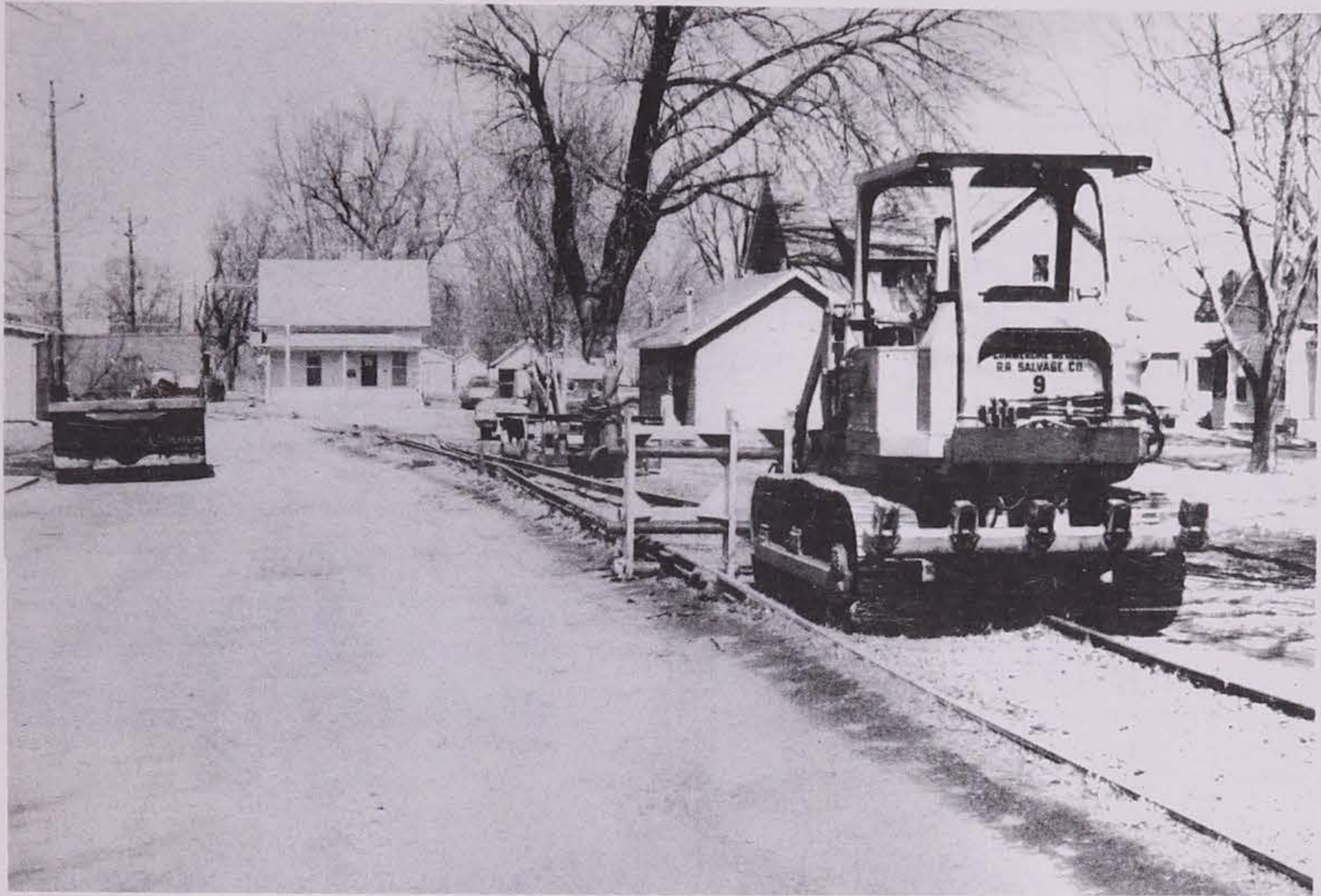
Track being removed on South 6th Ave. Washington. March 11, 1981.
