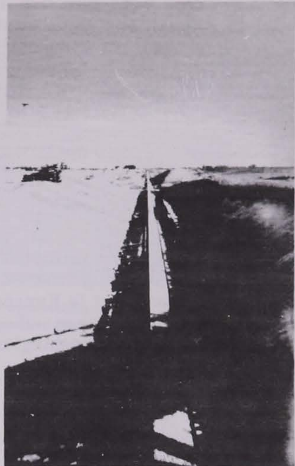
New Rock Island Cutoff from Coppock Road Bridge. May, 1947
