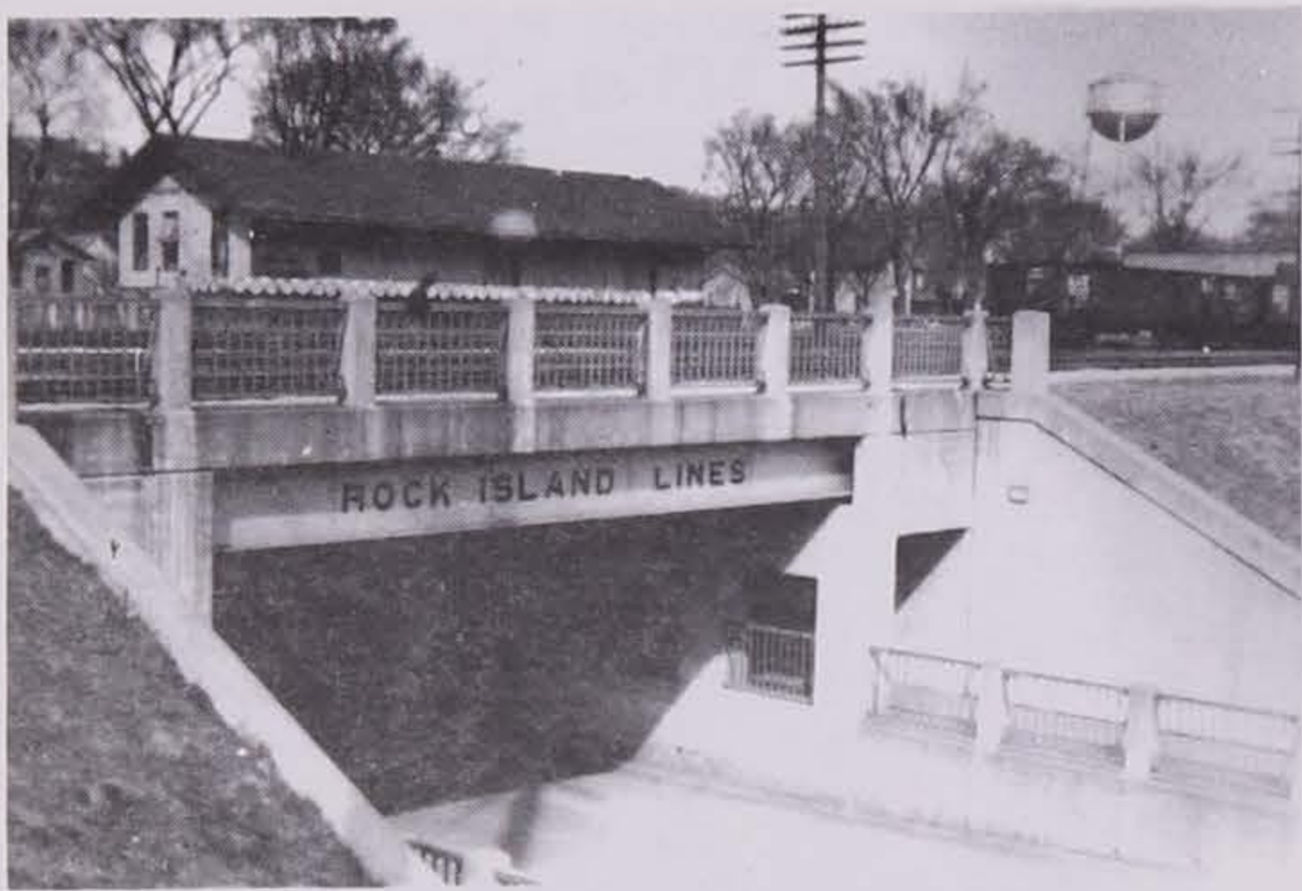
Rock Island - Milwaukee Road Underpass. Built in 1939 Milwaukee Freight Depot North Side of Tracks. March, 1945.
