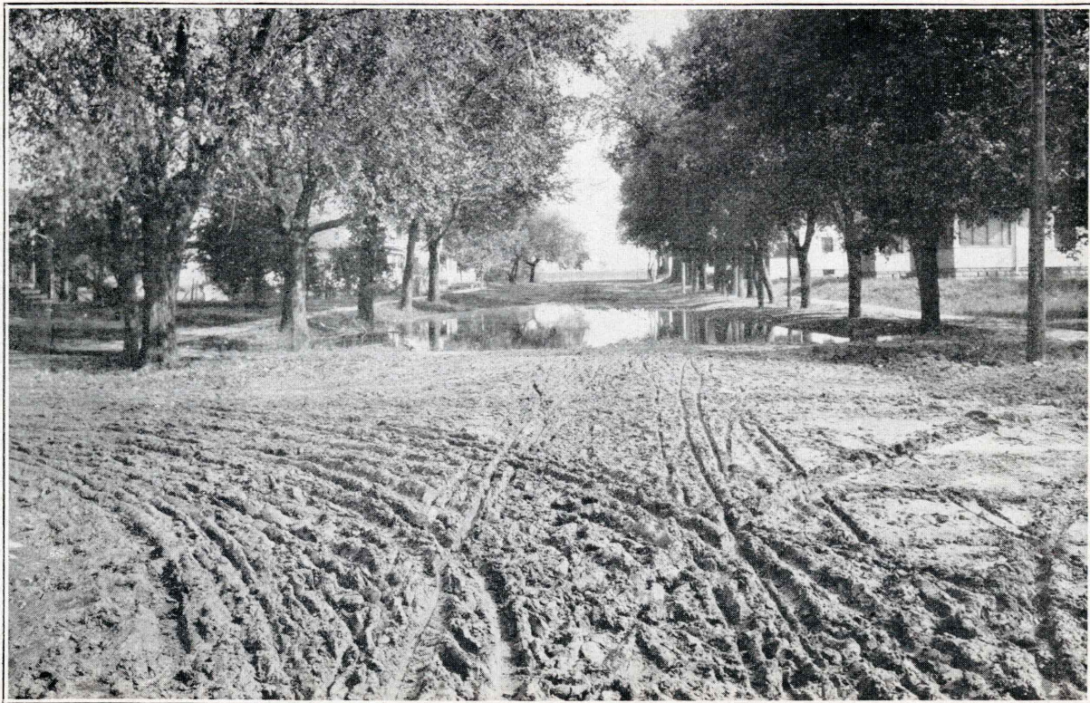
A street must be well drained before it is oiled. The street shown here would be little benefited by oiling.
