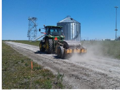
High-energy impact compaction
