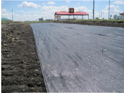
Woven geotextile over subgrade
