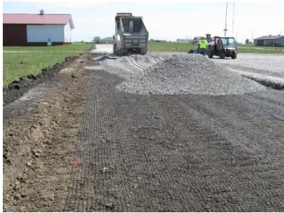
Biaxial geogrid over subgrade
