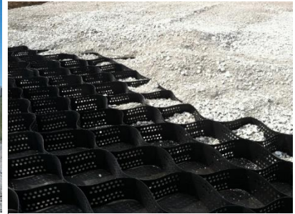
6 in. geocell over woven geosynthetic layer placed on subgrade
