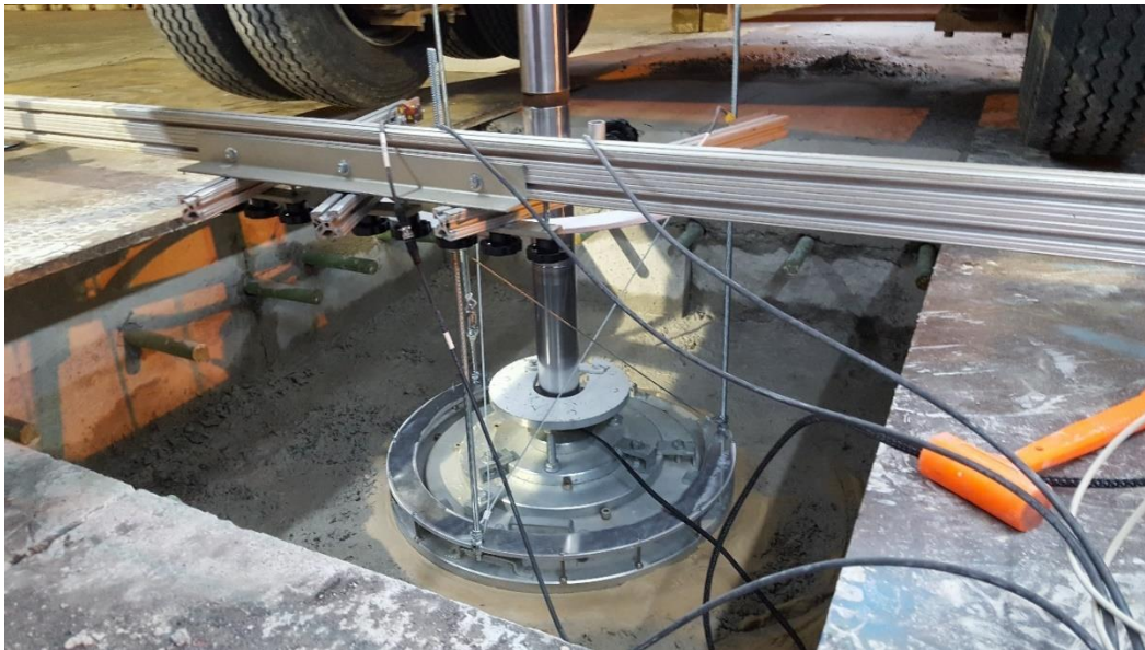
Figure 20. 30 in. diameter loading plate setup for static APLT to measure modulus of subgrade reaction values under an existing pavement in a core hole
