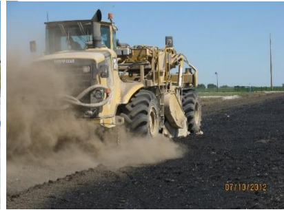
PC + Black MF-PP fiber stabilization of reclaimed subbase
