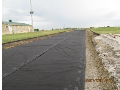
Nonwoven geotextile over subgrade
