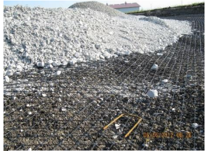
Triaxial geogrid placed over subgrade
