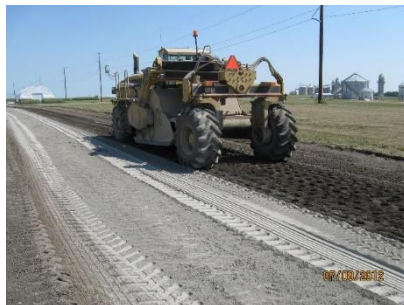
PC stabilization of reclaimed subbase
