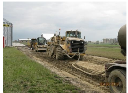
FA stabilization of subgrade
