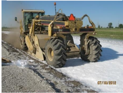
PC + White PP Fiber stabilization of reclaimed subbase
