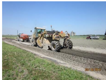
PC stabilization of subgrade
