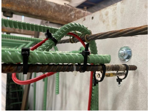
(b) Strain gauge at the top of a box girder
