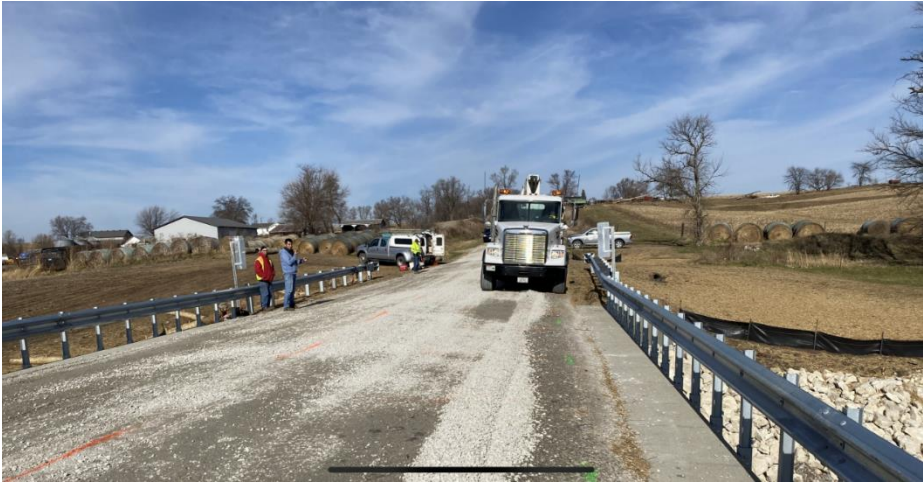
Figure 23. Live load test
