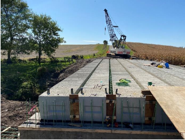
(a) Box girders placed
