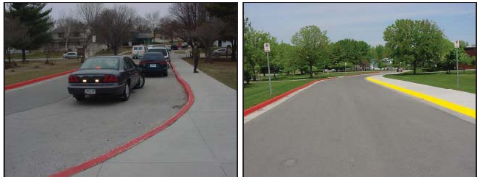
Figure 4.28. Confusing message sent by red fire lane marking (left) and modification to clarify the parking restrictions (right)
