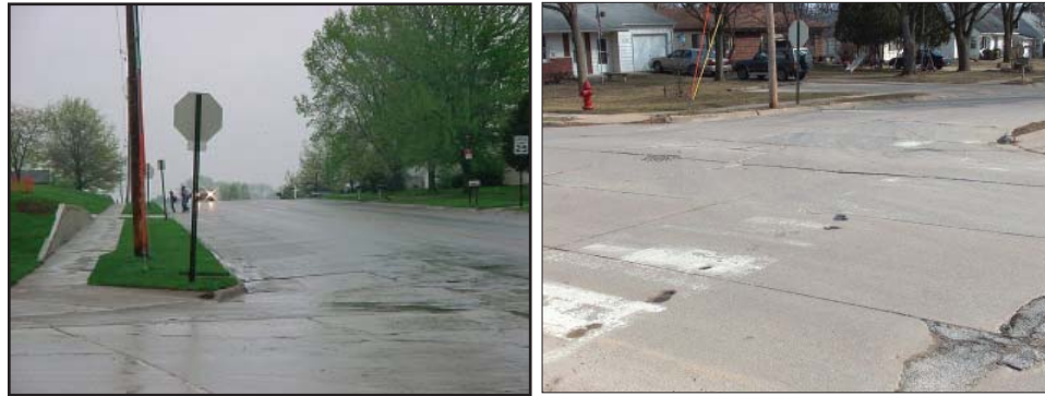
Figure 5.26. Poor and absent intersection crosswalk pavement marking
