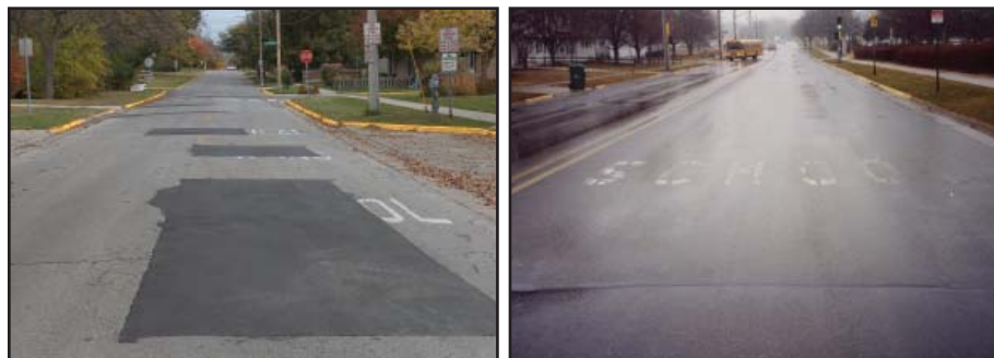
Figure 5.10. Obliterated and faded pavement markings
