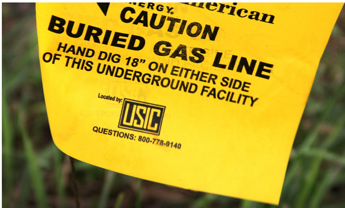
Iowa's One Call law requires marking of underground utility infrastructure at least 48 hours in advance of digging. A yellow locate flag indicates an underground natural gas pipeline.
