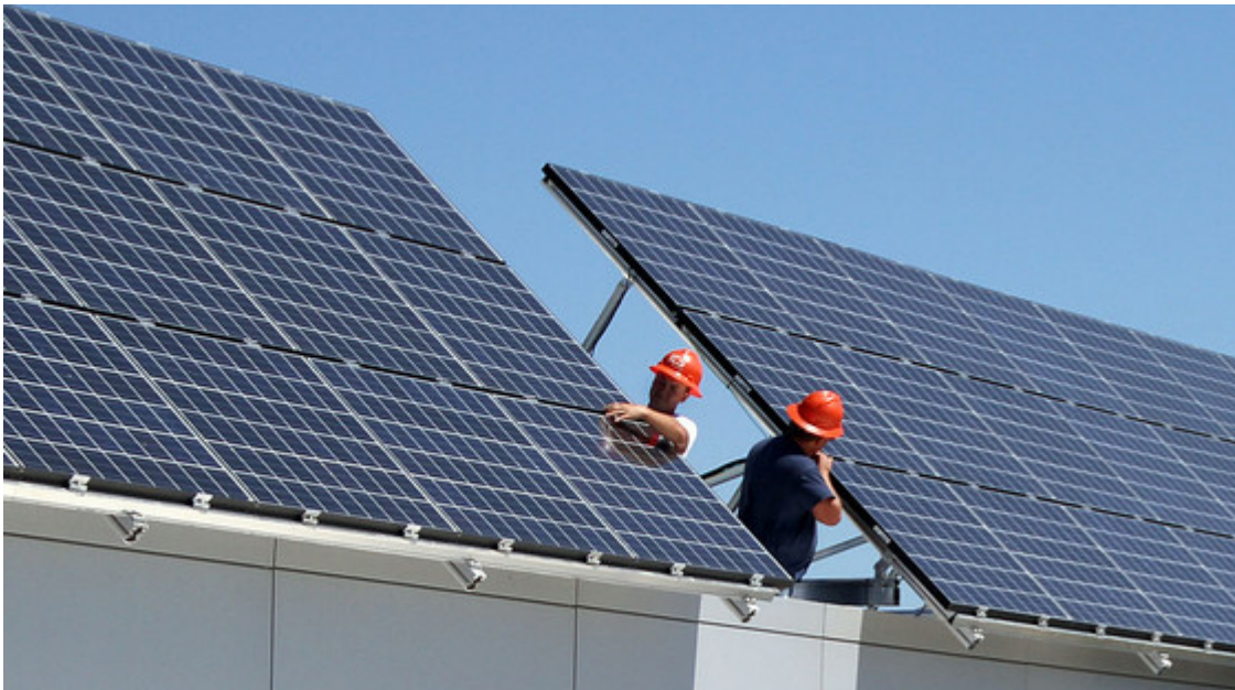
Construction workers adjust solar panels at a project in central Iowa.
