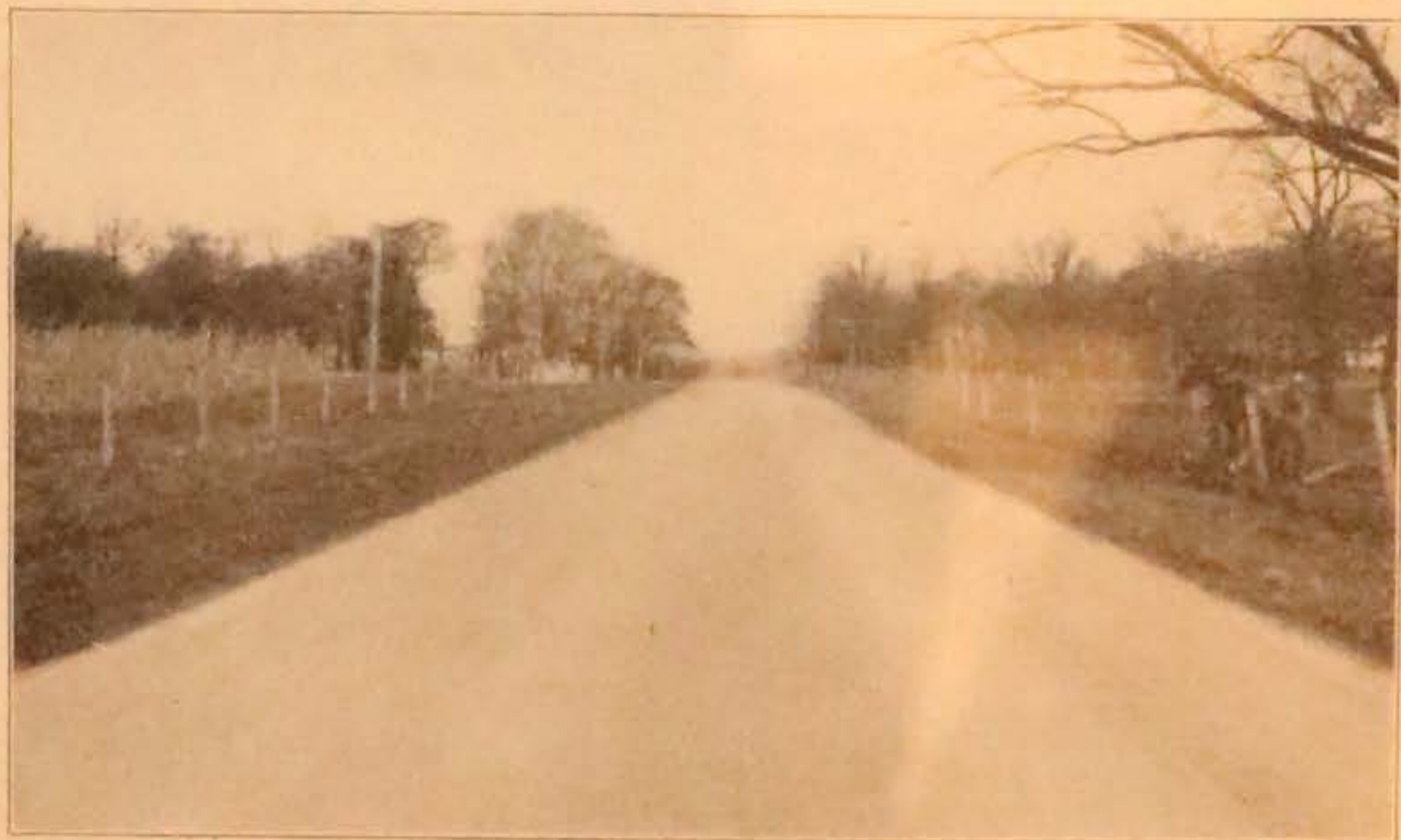
FIG. 80. This gravel road in Greene County is another kind of good road and serves very well where gravel is plentiful. What is done to the road before the gravel is put on?
