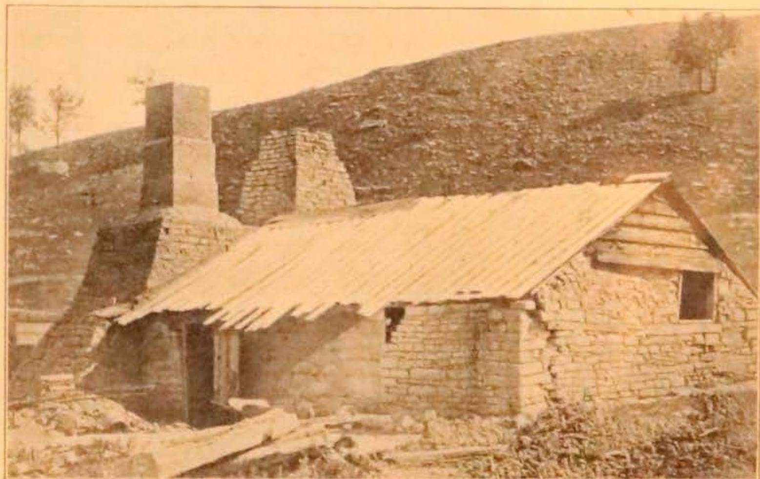
FIG. 8. Water's old lead smelter near Dubuque is said to have been the earliest smelter built in Iowa. Notice the great limestone bluff and the limestone used in the building
