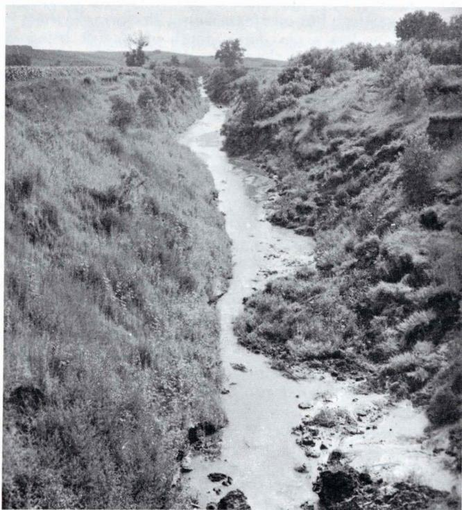
Figure 26.—Top, upstream view of the Willow drainage ditch less than a year after construction (1920-1921) in sec. 3, T. 81 N., R. 42 W., Harrison County, Iowa; depth 11 feet. (Photo by courtesy of H. D. Smith, Woodbine, Iowa.) Bottom, upstream view of the ditch in 1957; depth 42 feet.
