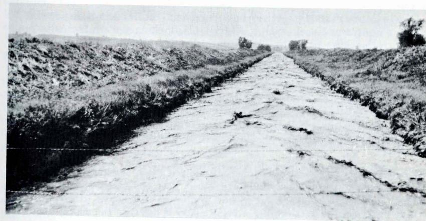
Figure 29.—Willow drainage ditch in sec. 9, T. 81 N., R. 42 W., Harrison County, Iowa, at nearly bank-full stage in 1920, shortly after construction. Note turbulence of the water surface; depth of flow is approximately 10 feet. (Photograph by courtesy of H. D. Smith, Woodbine, Iowa.)
