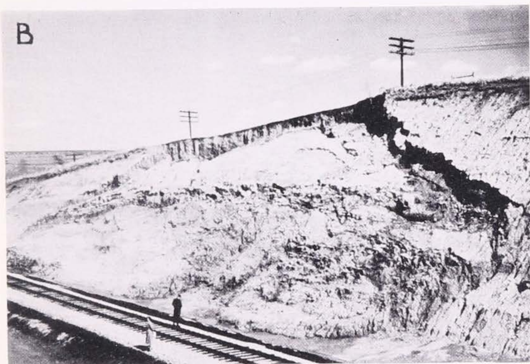
FIGURE 4.—Earthslide in cut 31, September 1953 (A) and April 1954 (B).
