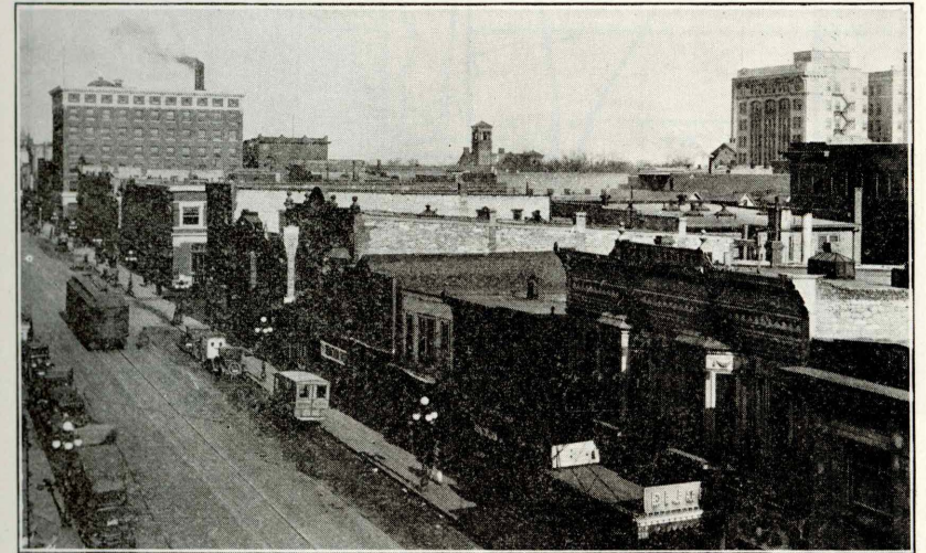
Fig. 15. Looking north along Federal Avenue.
