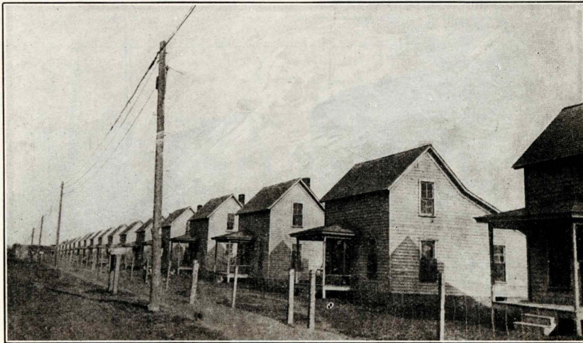
Fig. 49. The workmen's houses provided by the Northwestern States Portland Cement Company. See Fig. 68 for their position relative to the cement plant.
