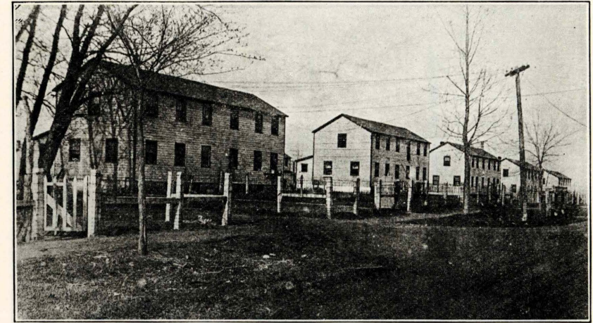
Fig. 48. Industrial housing furnished by the Lehigh Portland Cement Company.
