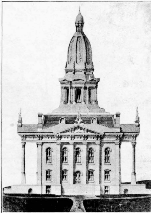
DES MOINES SECOND COURT HOUSE Torn down to make place for the new court house
