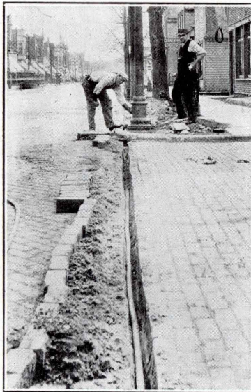
CROSSING BRICK PAVEMENT WITH CABLE
