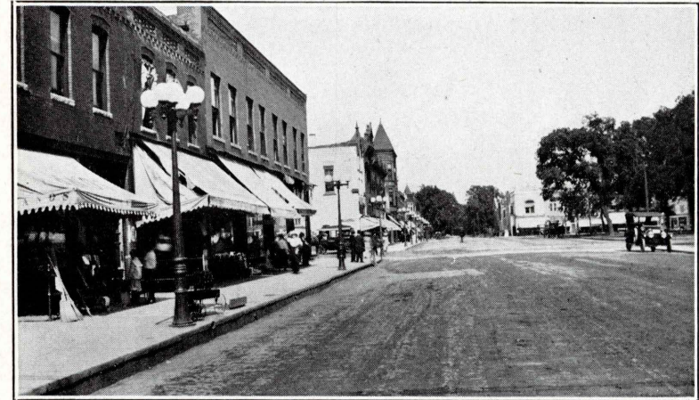
FIVE LIGHT POSTS IN USE AT FAIRFIELD, IOWA
