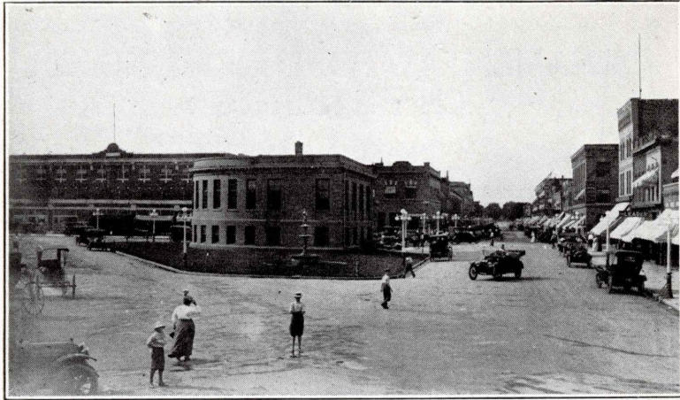
ORNAMENTAL POST LIGHTING, PERRY, IOWA
