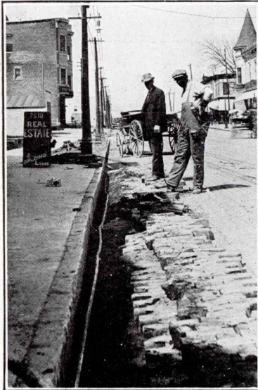
LAYING CABLE OUTSIDE OF CURB
