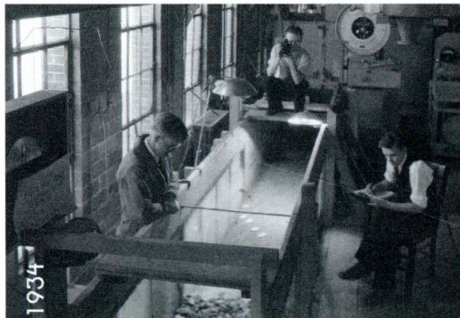
mississippi river lock and dam model, sponsor: u.s. army corps of engineers
