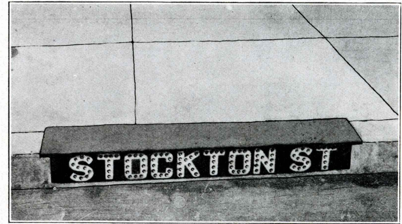
Fig. 13.—An illuminated street-name sign set in the curbing.
