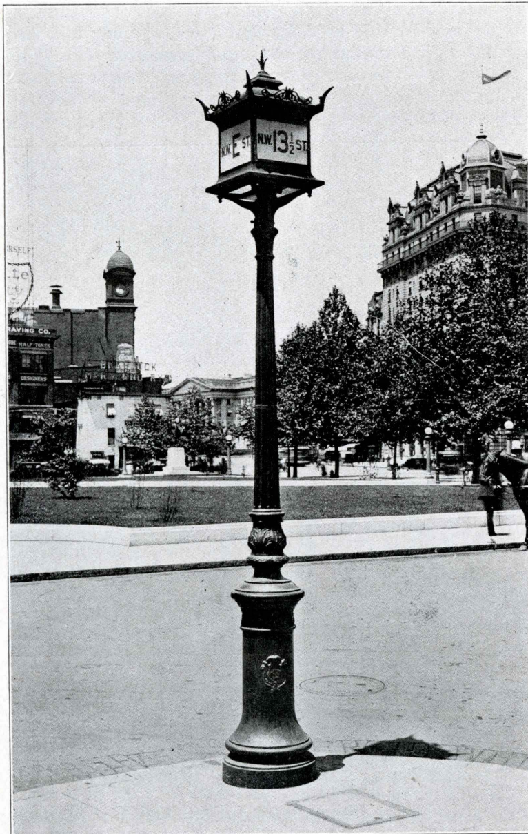
Fig. 18.—The lantern type of street-name sign used at the more important street intersections in Washington, D. C.
