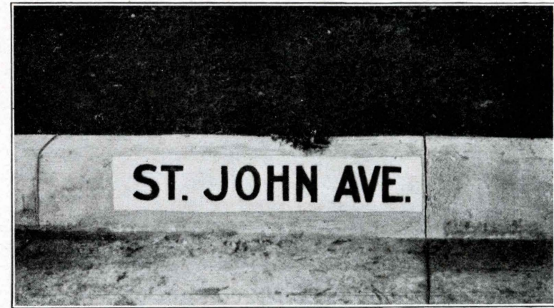
Fig. 11.—A street-name sign painted on the vertical face of the concrete curbing. Black letters on a white ground.
